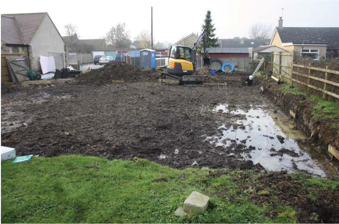
Plate 1. General view of site looking south.
