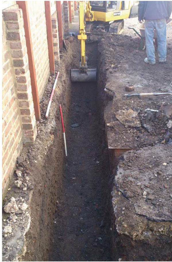
Plate 1. Footing trench, looking east, Scale: 1m.
