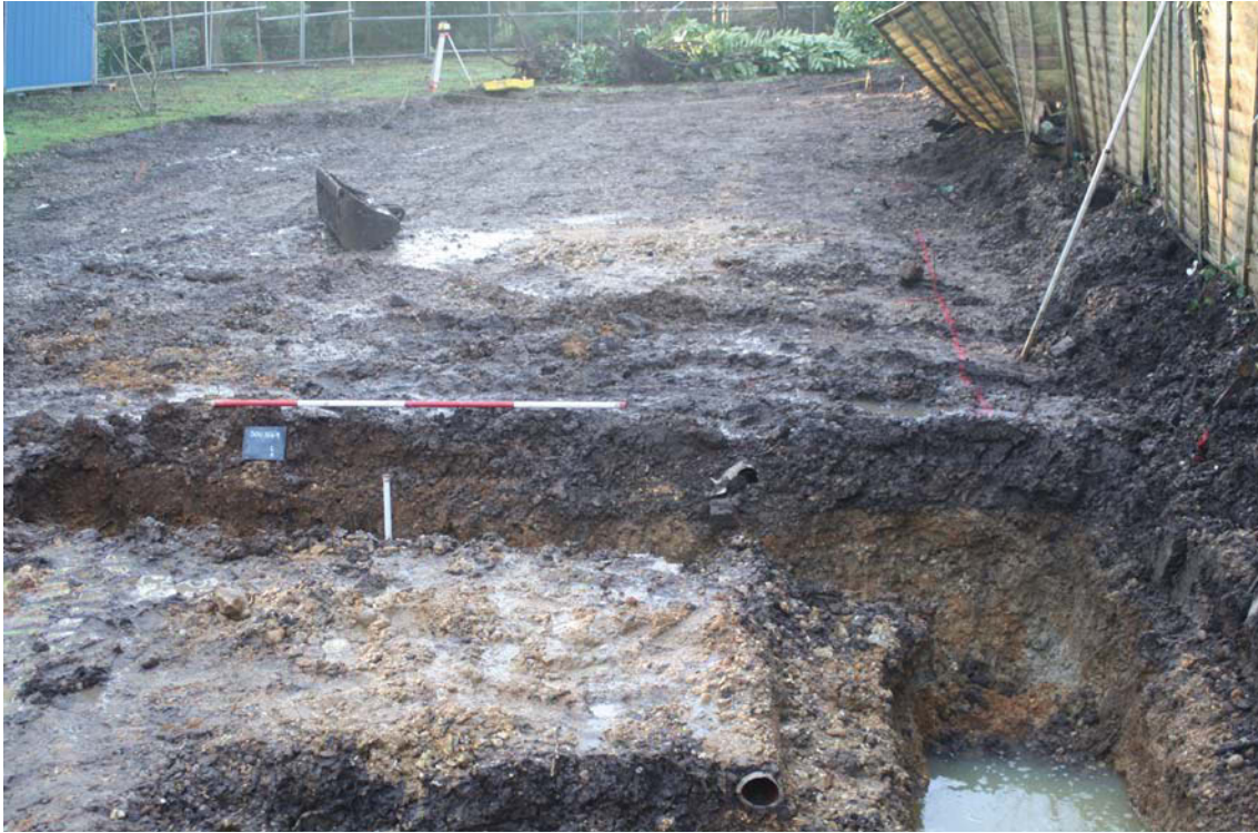
Plate 1. Footing trenches under excavation, looking south, Scale: 2m.
