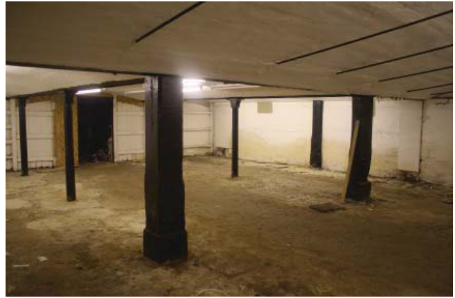
Plate 8. Interior, general view of room E, looking south.
