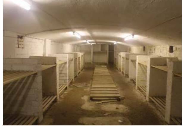
Plate 6. Interior, general view of room D, looking north west.
