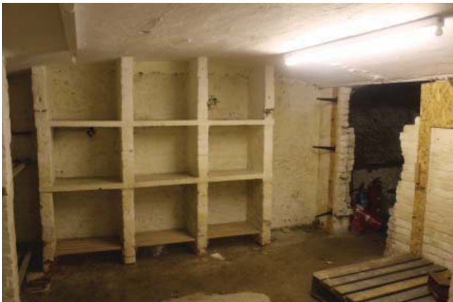
Plate 7. Interior, general view of room D, looking south.
