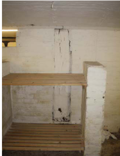
Plate 14. Interior, room D, timber post in dividing wall, looking north west.
