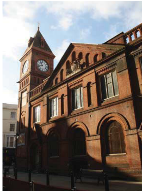
Plate 2. Exterior, east elevation, looking south west.
