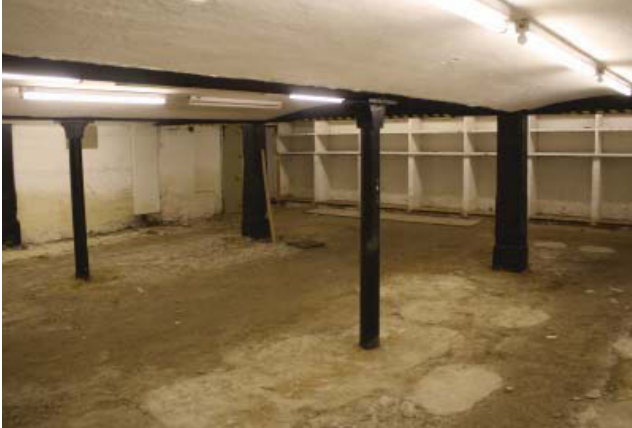
Plate 9. Interior, general view of room E, looking west.
