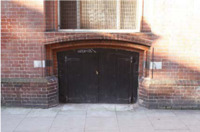
Plate 1. Exterior, entrance leading to vaults, looking north west.
