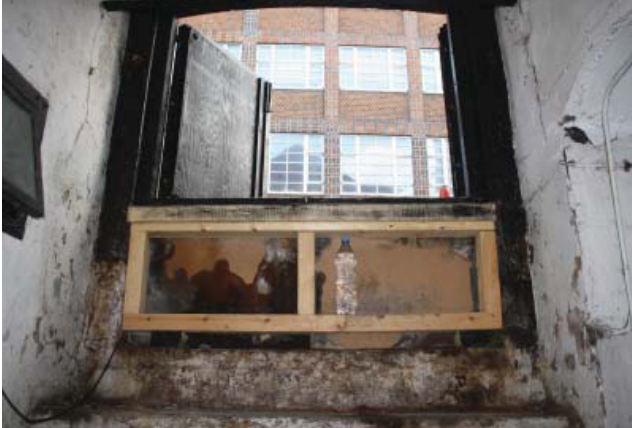
Plate 13. Interior, room A, close-up of entrance into vaults, looking south east.
