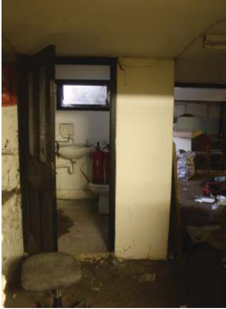
Plate 5. Interior, room A, looking south west towards room C.
