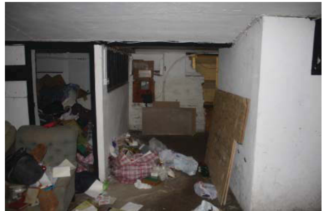
Plate 4. Interior, general view of room A, looking north east.
