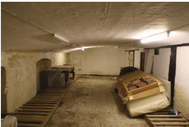
Plate 11. Interior, general view of room F, looking north west.
