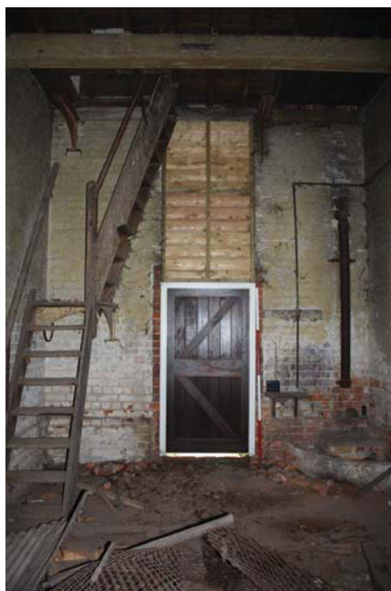
Plate 9. Stairs in room 2, looking North, Scale: 2m.
