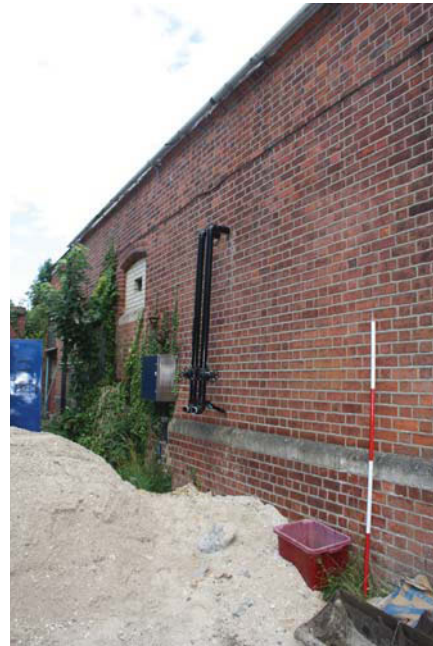
Plate 14. Pump house (West elevation), looking Northeast, Scale: 2m.
