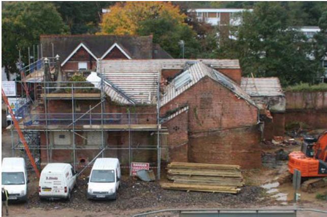
Plate 13. Pump house (East elevation), looking West.
