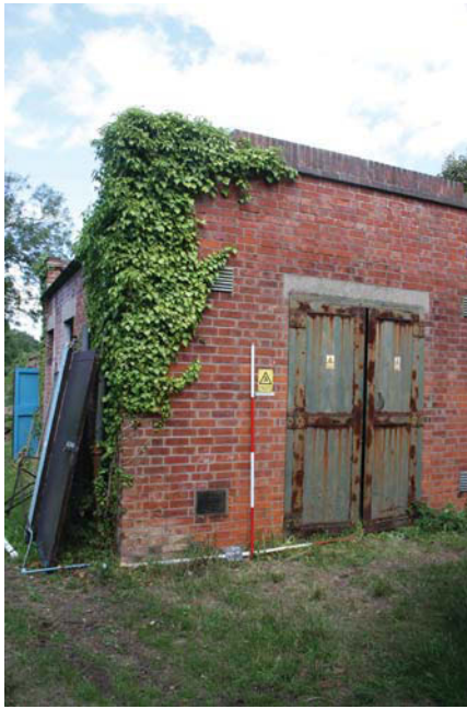
Plate 21. Substation, looking Northeast, Scales: 2m and 1m.
