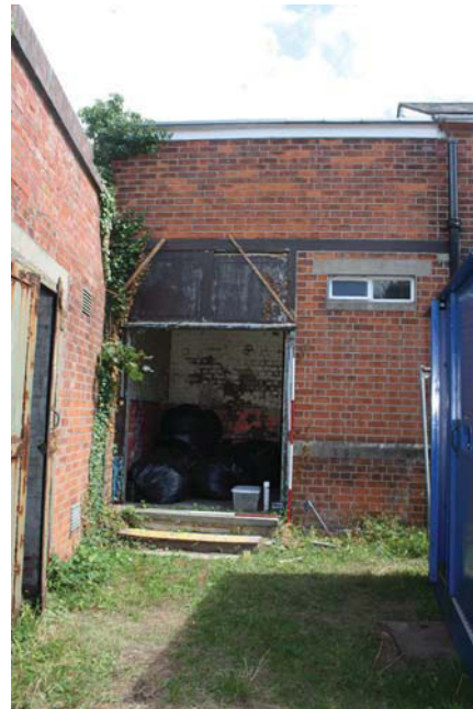
Plate 20. Former substation, looking East, Scales: 2m and 1m.
