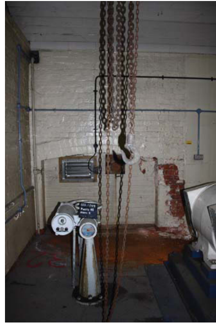
Plate 16. Blocked door in room 8, looking West.
