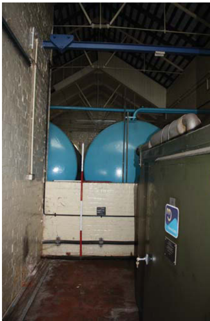
Plate 19. Room 11, looking South, Scales: 2m and 1m.
