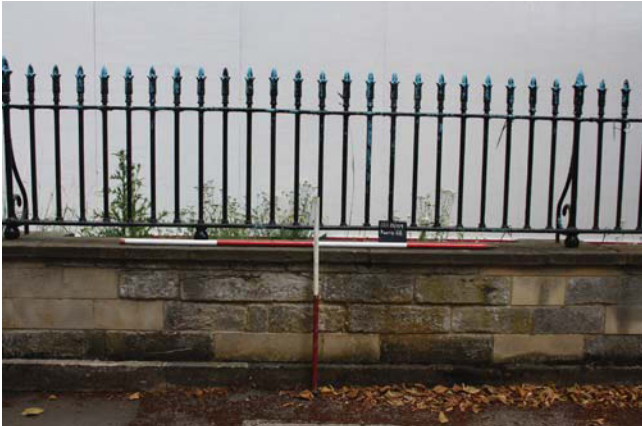
Plate 1. Boundary wall, looking North, Scales: 2m and 1m.
