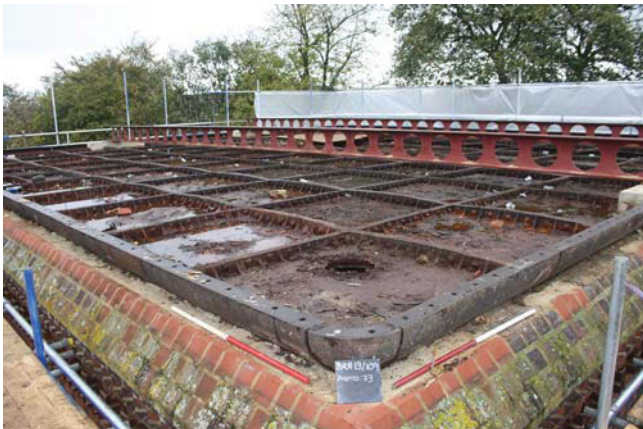
Plate 7. The roof, looking Northeast, Scales: 1m.
