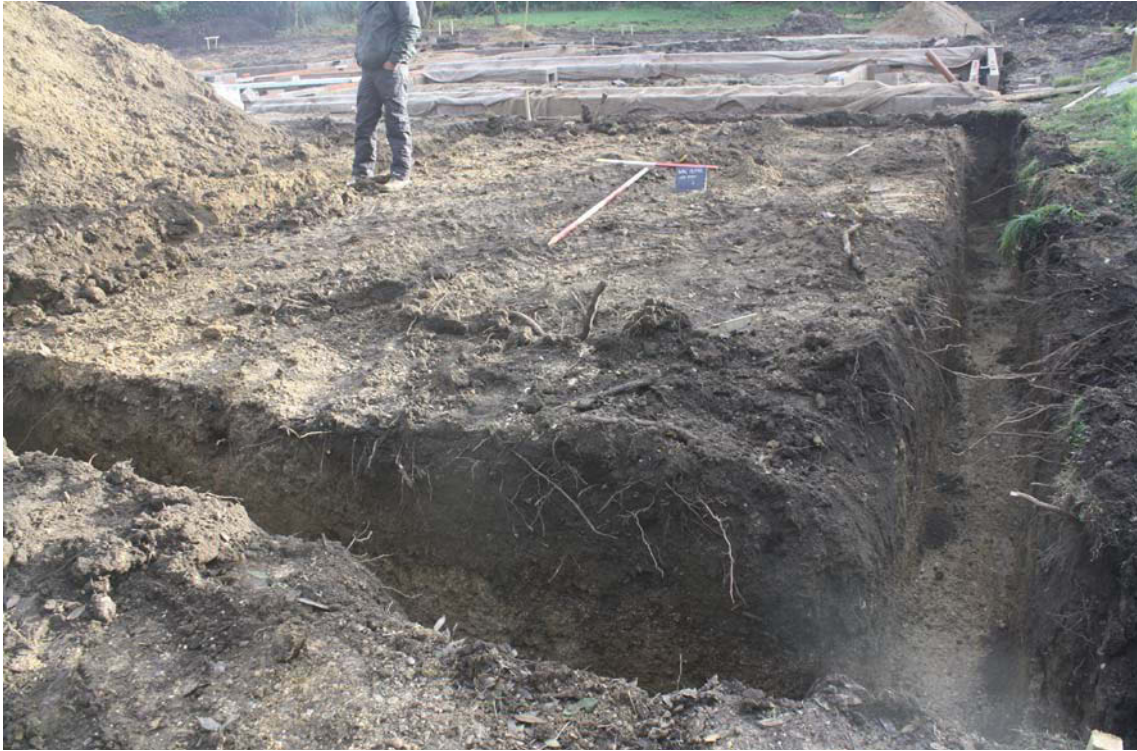
Plate 1. Garage foundation, looking south, Scales: 2m and 1m.
