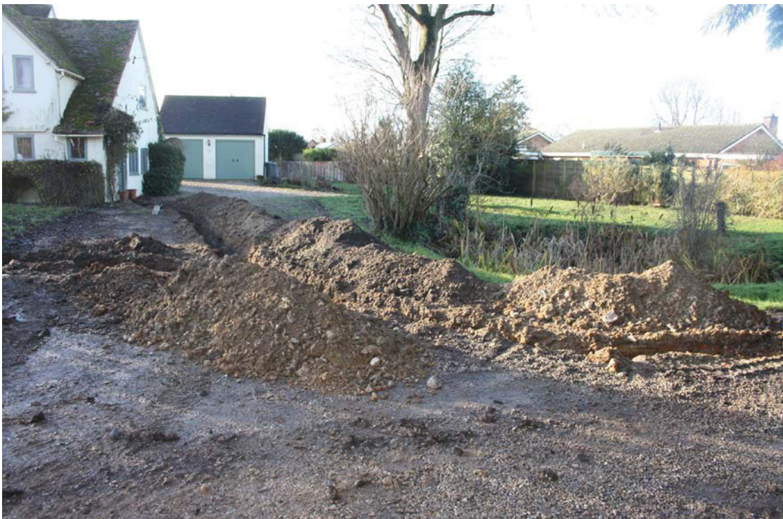
Plate 2. Service trench, looking west.
