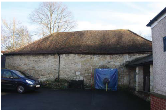
Plate 3. Blocked cart door, looking East, Scales: 2m and 1m.
