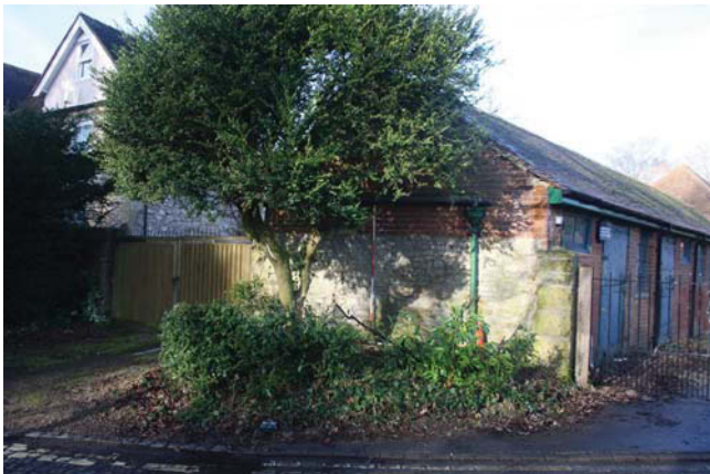
Plate 11. South wall of the stable block, looking Northwest, Scales: 2m.
