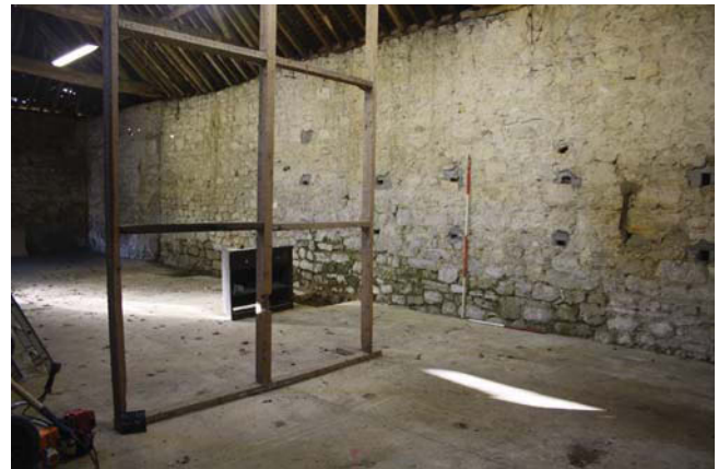
Plate 8. West wall of barn, looking Southwest, Scales: 2m and 1m.
