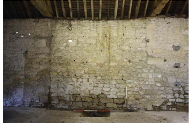
Plate 6. Blocked cart door, looking West, Scales: 2m and 1m.
