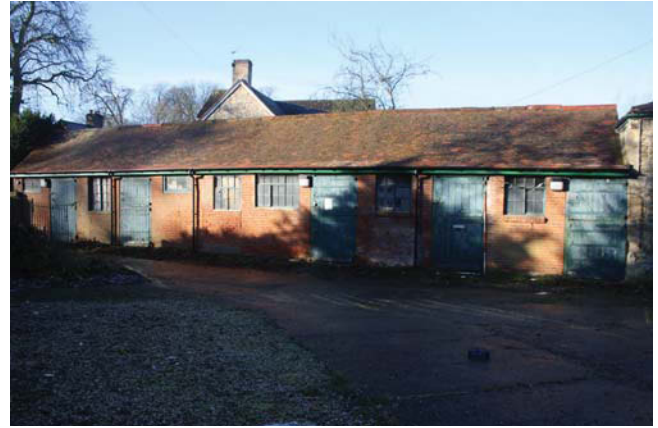
Plate 10. The stable block, looking Southwest, Scales: 2m and 1m.
