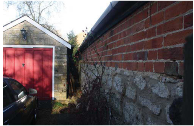
Plate 12. West wall of stable block, looking North.
