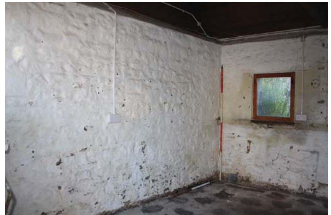
Plate 14. View to window, looking Southwest, Scales: 2m and 1m.
