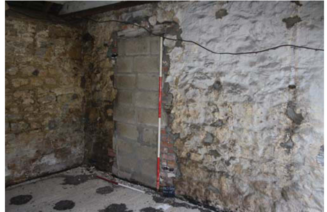
Plate 2. Blocked door, looking Northwest, Scales: 2m and 1m.
