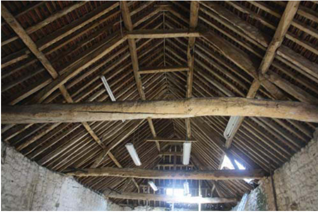
Plate 9. Barn roof trusses, looking North.
