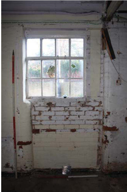
Plate 13. Blocked stable door, looking East, Scales: 2m and 1m.
