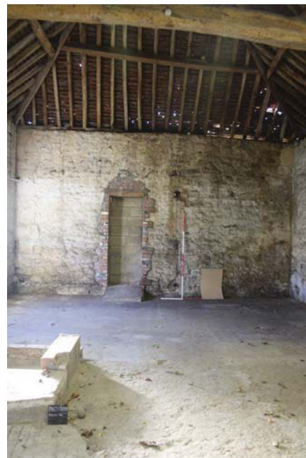
Plate 4. South wall of barn, looking South, Scales: 2m and 1m.
