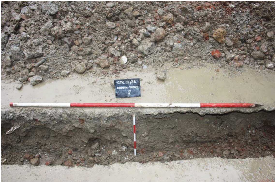
Plate 2. Representative section of pipe trench, looking north, Scales: 2m and 1m.
