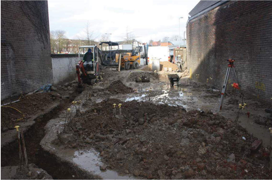
Plate 1. Excavation of pipe trenches in progress, looking north.
