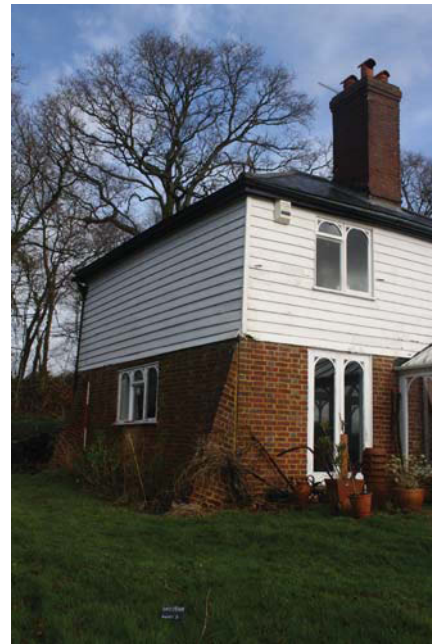
Plate 4. South and West elevations, looking North east, Scales: 2m and 1m.
