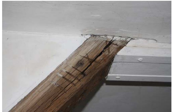
Plate 6. Carpenters mark in room 10, looking South.
