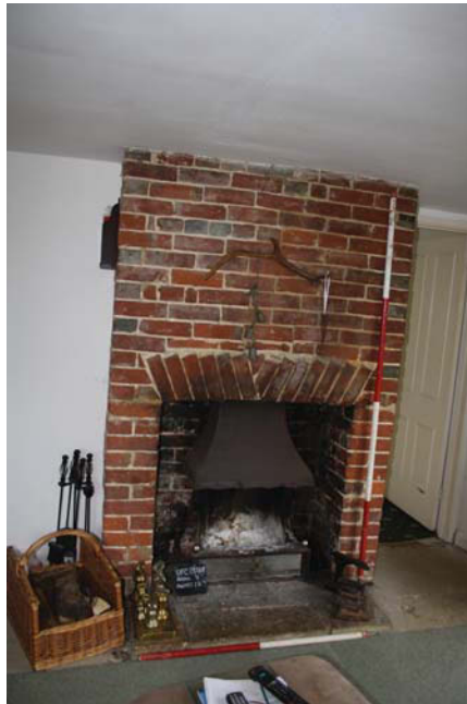
Plate 9. Fireplace in room 7, looking East, Scales: 2m and 1m.
