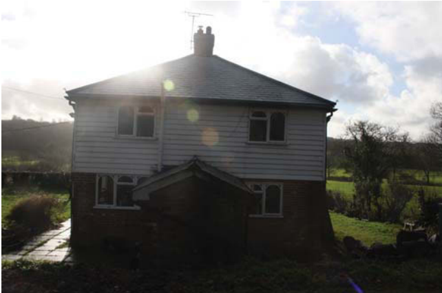
Plate 1. North elevation, looking South, Scales: 2m and 1m.
