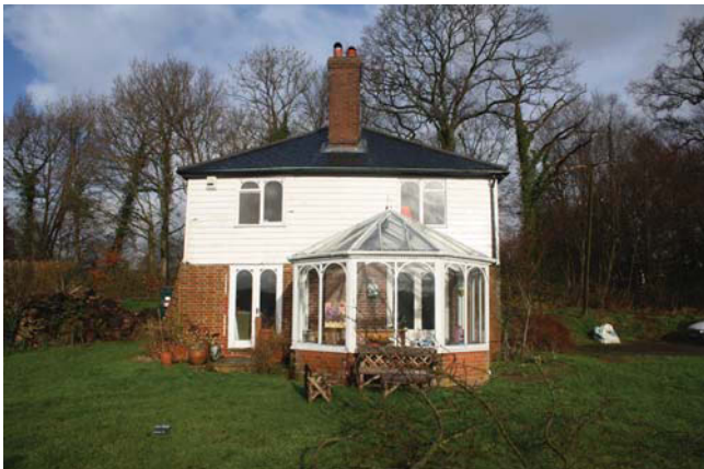
Plate 3. South elevation, looking North, Scales: 2m and 1m.
