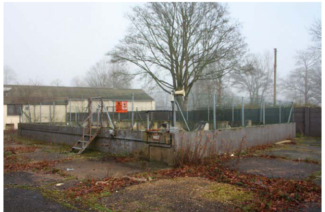
Plate 24. Tank 1407, looking northeast.
