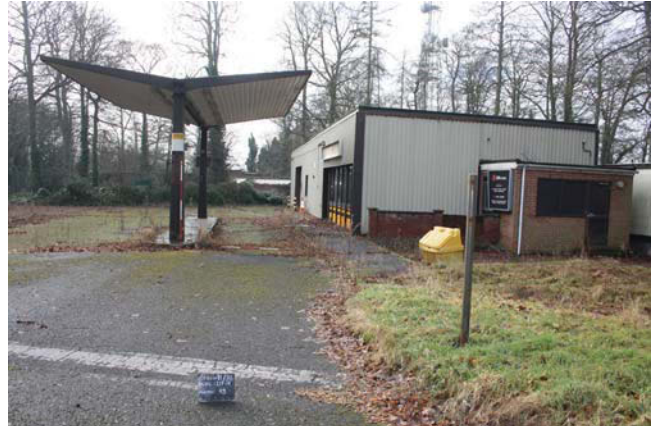
Plate 18. Garage, looking southwest, scales: 2m.
