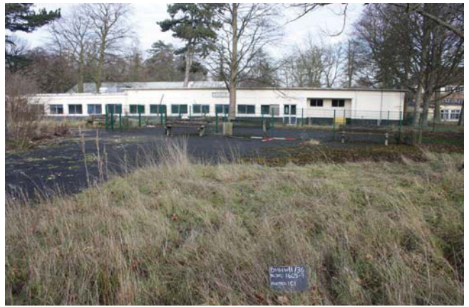
Plate 32. Cafeteria, looking northeast, scales: 2m.
