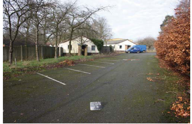
Plate 10. Prefabricated huts, blocks 1101 and 1102, looking northwest, scales: 2m.
