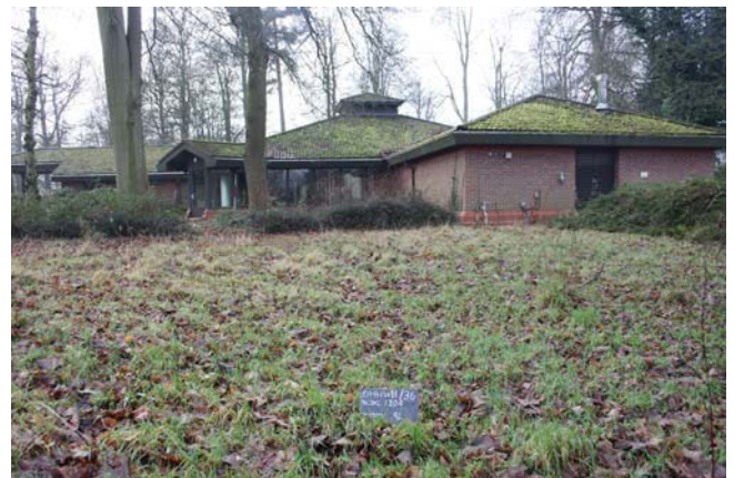
Plate 16. Block 1204, looking southwest, scale: 2m.
