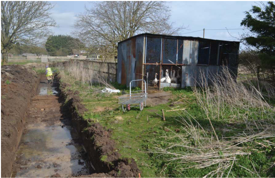
Plate 3. General view of Trench 11 looking north
