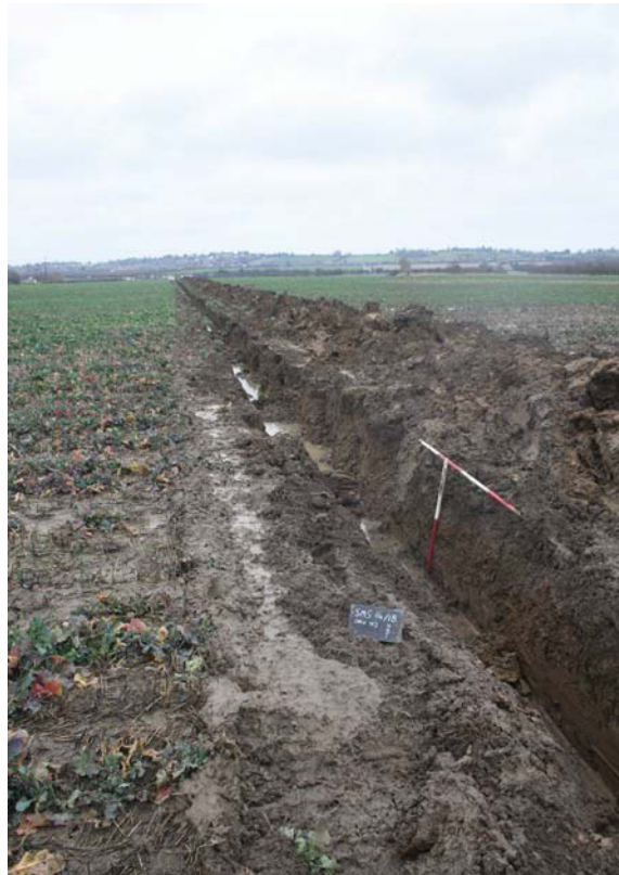
Plate 1. High voltage cable trench 2, looking north, Scales: 2m and 1m.
