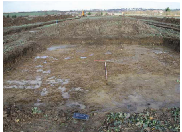
Plate 3. Substation strip, looking west, Scales: 2m and 1m.
