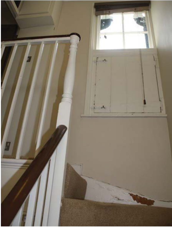
Plate 17. Landing S8 looking south from stairwell
