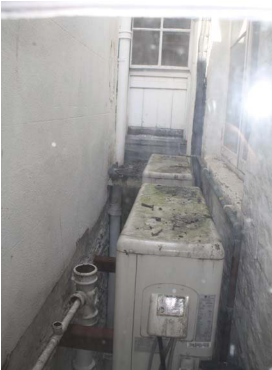
Plate 23. Exterior, rear lightwell looking north
