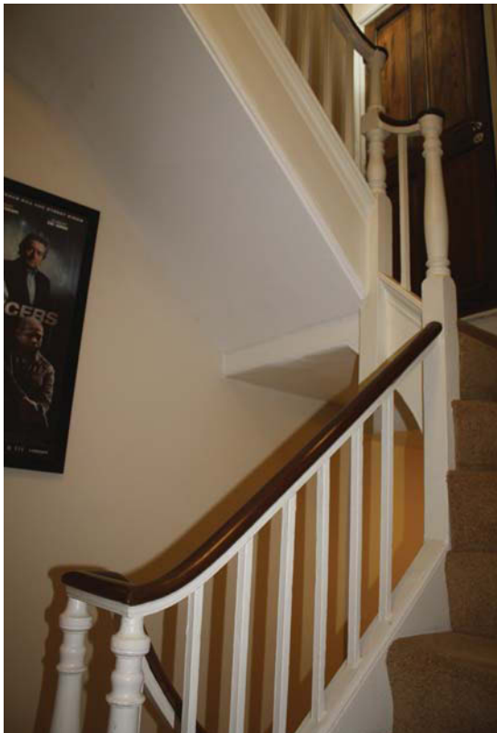
Plate 15. Northern staircase looking north-west from F6
