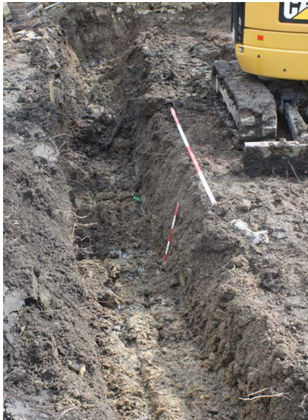
Plate 2. New footing trench, looking west, Scales: 2m and 1m.
