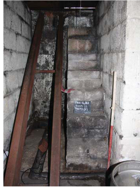
Plate 6. Interior, room 11, access and loading ramp, looking south east, Scale: 1m
