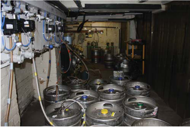
Plate 5. Interior, room 11, north west wall.
