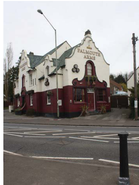
Plate 2. Exterior, south elevation with street entrance, looking north.
