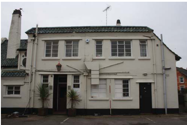
Plate 3. Exterior, rear elevation, looking south west, Scale: 2m.
