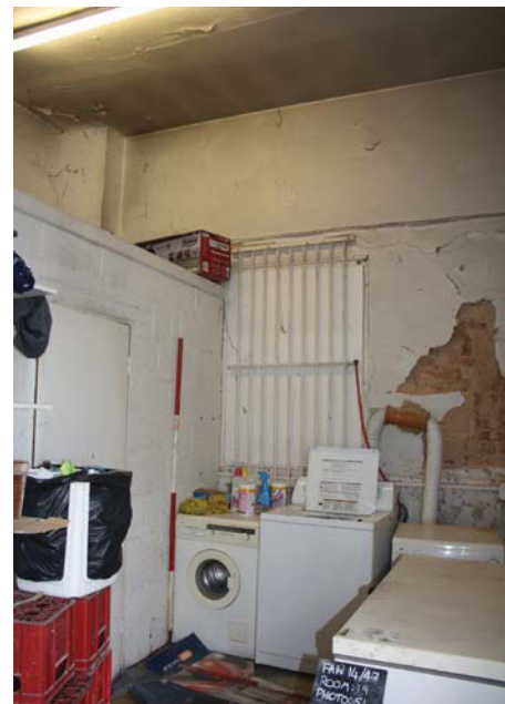
Plate 24. Interior, room 19 south corner, Scale: 2m.
