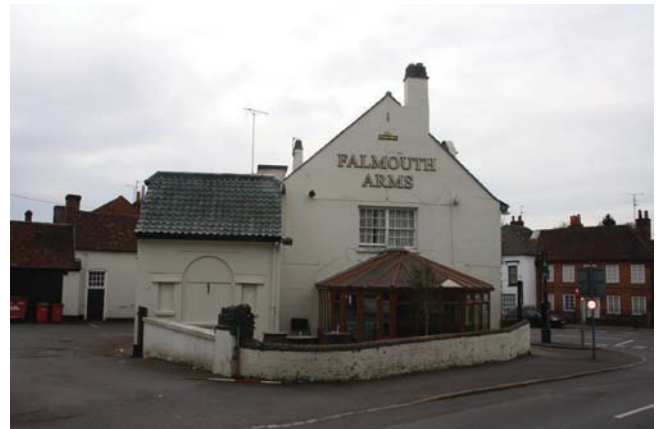
Plate 4. Exterior, north elevation with conservatory, looking south, Scale: 2m
