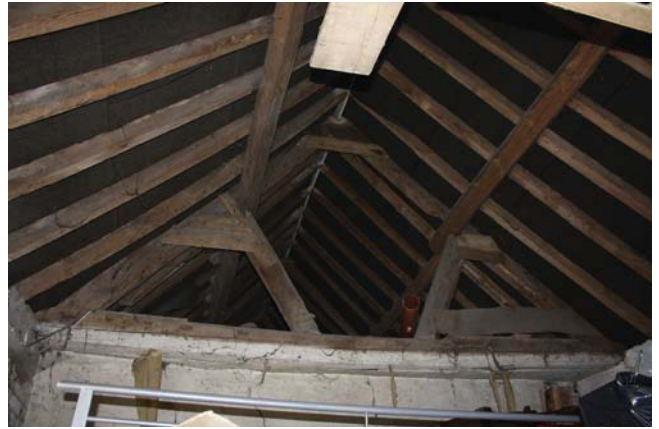
Plate 28. Interior, room 20 central truss, looking north east.
