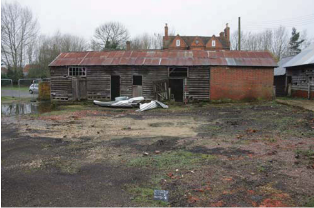
Plate 41. Exterior, east elevation of Unit F, Scales: 2m and 1m.
