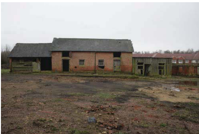
Plate 23. Exterior, north elevation of Unit C, Scales: 2m and 1m.
