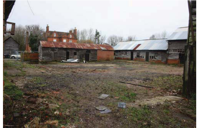
Plate 2. Exterior, courtyard area, looking north west, Scale: 2m.
