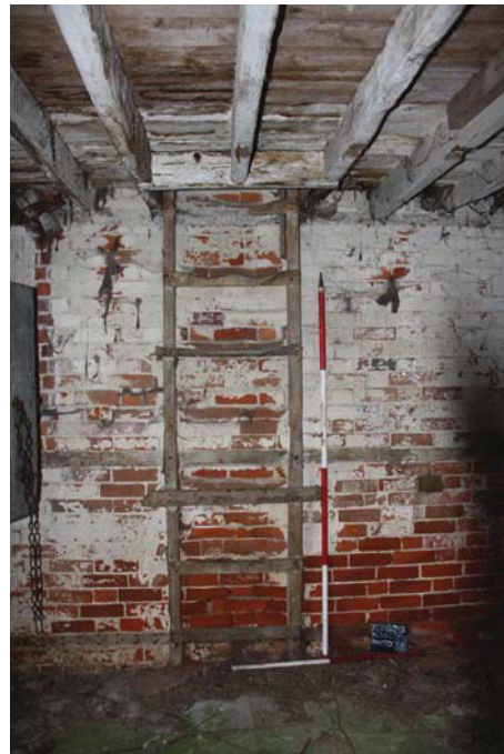
Plate 30. Interior, access stairs to hayloft of west wall, Scales: 2m and 1m.
