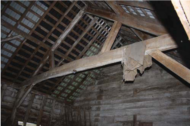
Plate 5. Interior, east wall and roof trusses.
