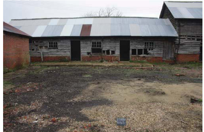
Plate 6. Exterior, south elevation of Unit A, Scales: 2m and 1m.
