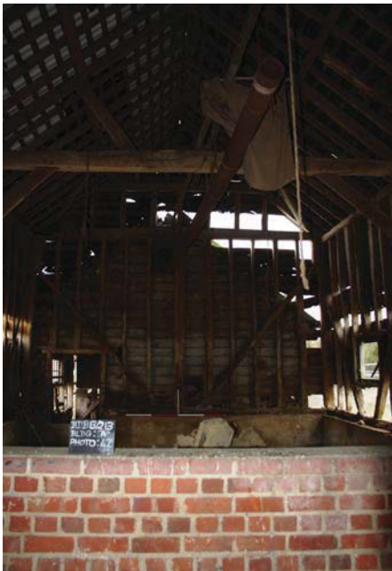
Plate 11. Interior, Unit A, looking east, Scales: 2m and 1m.
