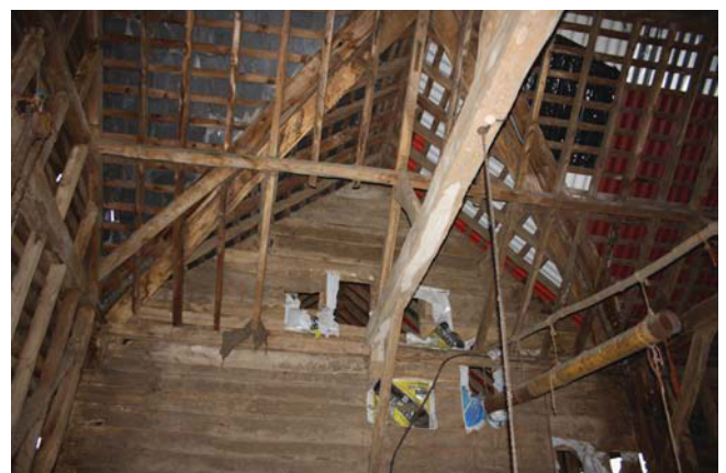
Plate 16. Interior, connecting wall of Unit B, looking south.
