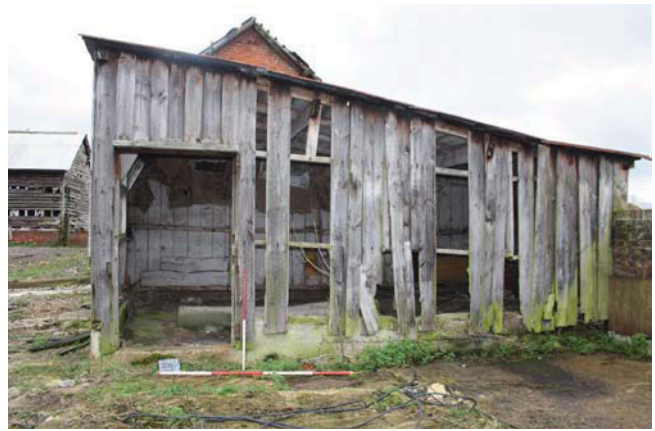
Plate 32. Exterior, west elevation of Unit C, Scales: 2m and 1m.
