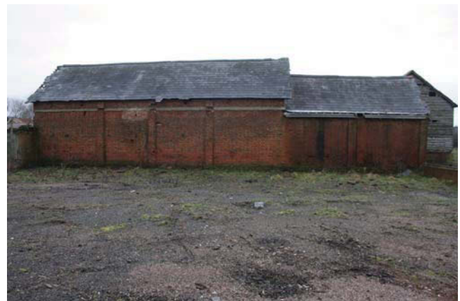
Plate 24. exterior, south elevation of Unit C.
