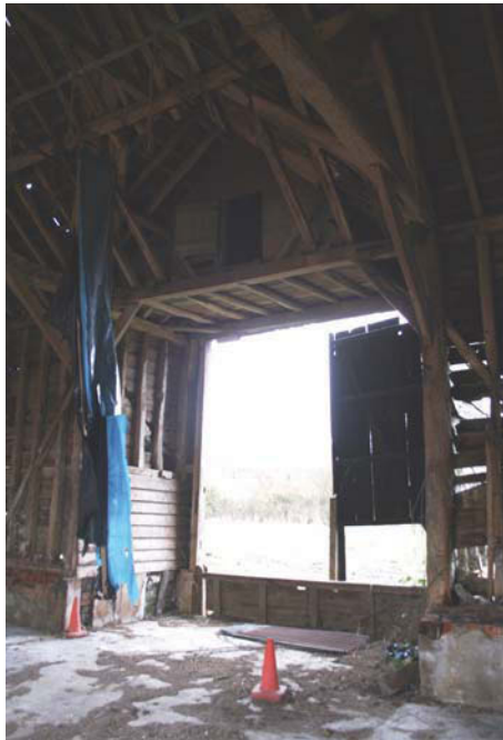
Plate 21. Interior, Unit B, cart shed door on west face.
