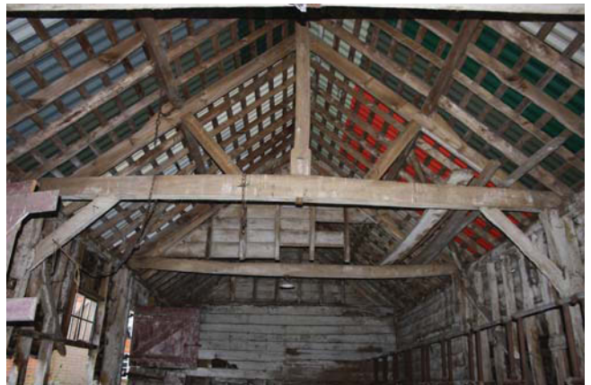
Plate 8. Interior, Unit A, trusses 1 and 2, looking west.
