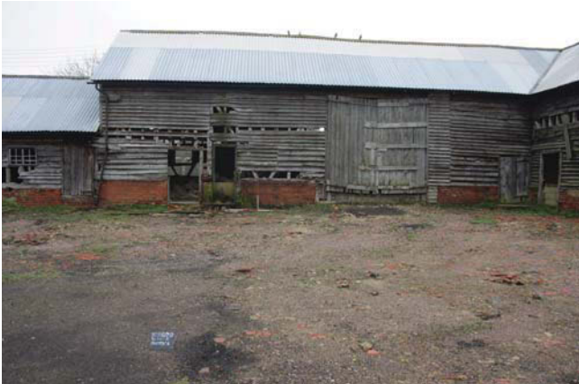
Plate 9. Exterior, south elevation of Unit A, Scales: 2m and 1m.
