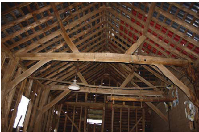
Plate 15. Interior, truss at east end of Unit A, looking east.
