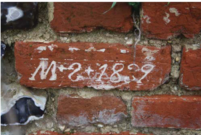
Plate 39. Exterior, Unit D, dated brick. looking east
