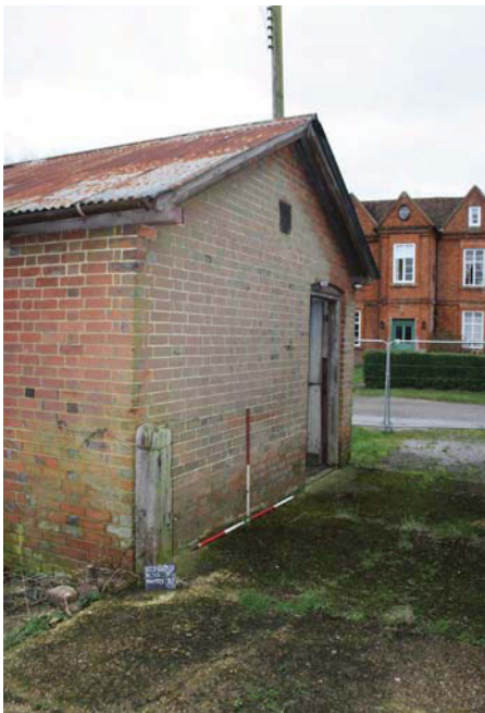
Plate 43. Exterior, Unit F, looking south west, Scales: 2m and 1m.
