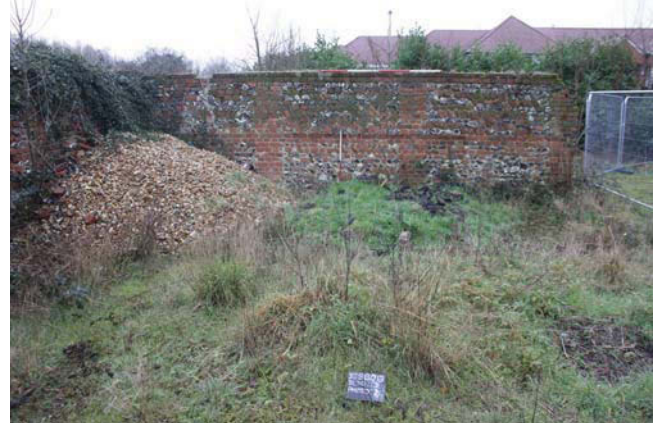
Plate 38. 'Interior' of Unit D, looking south, Scale: 1m.
