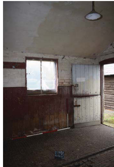
Plate 44. Interior, Unit F, looking north west, Scales: 2m and 1m.
