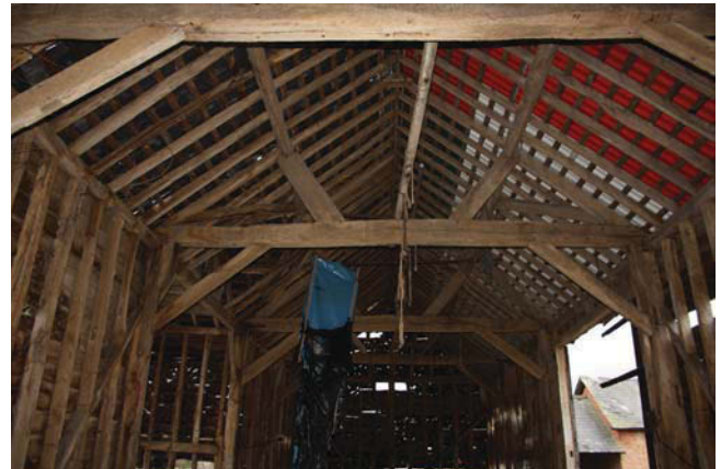
Plate 22. Interior, central truss of Unit B, looking south.
