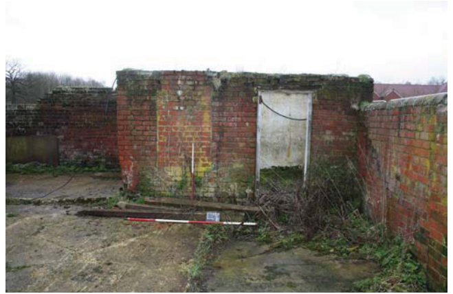
Plate 34. Exterior, north elevation of Unit D, Scales: 2m and 1m.
