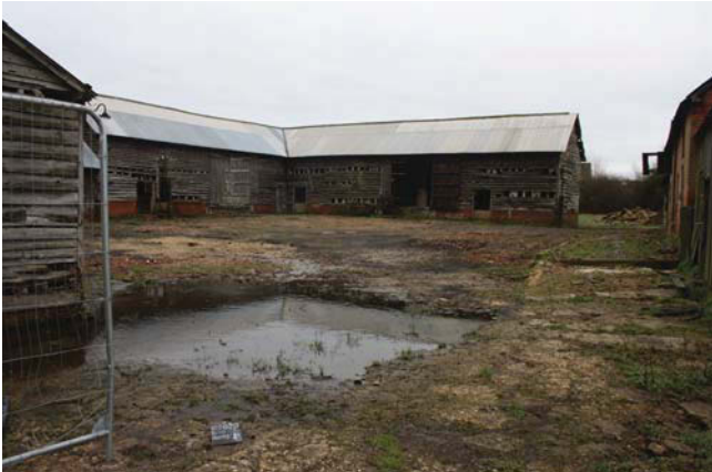
Plate 1. Exterior, courtyard area, looking north east, Scale: 2m.
