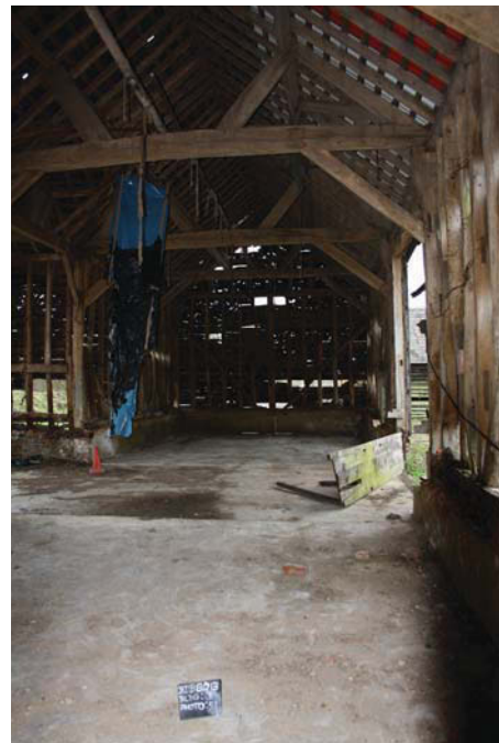
Plate 20. Interior, Unit B, looking south.
