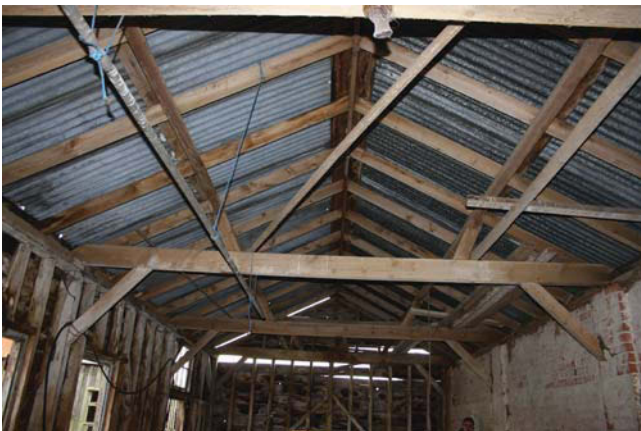
Plate 47. Interior, Unit F, central truss, looking south.
