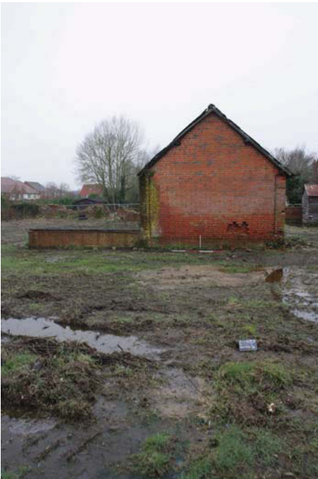
Plate 27. Exterior, east elevation of Unit C, Scales: 2m and 1m.
