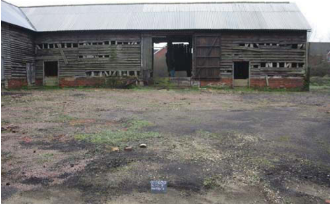
Plate 17. Exterior, west elevation of Unit B, Scales: 2m and 1m.
