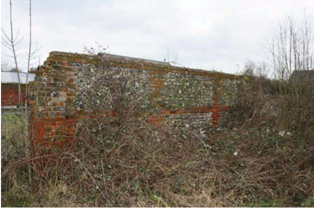
Plate 37. Exterior, Unit D, looking north east.
