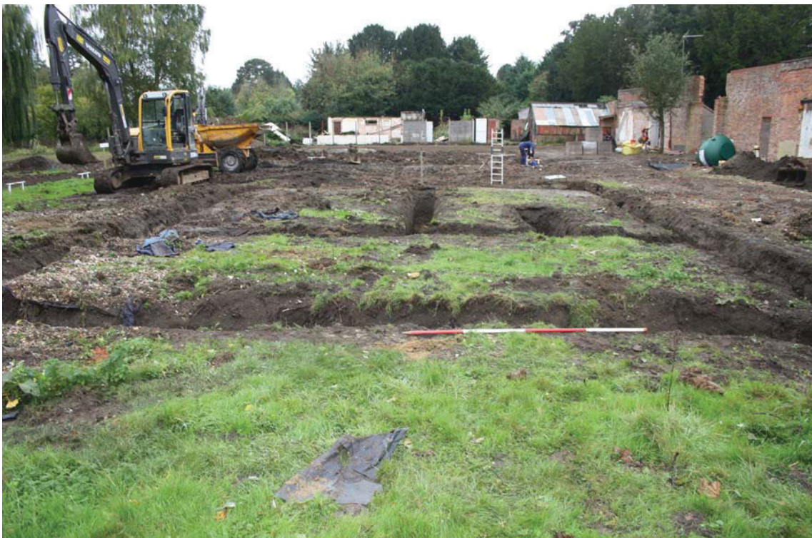
Plate 2. Plot 3 foundations looking South West. Scale 2m.
