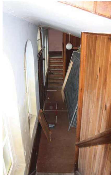
Plate 12. Interior, front entrance lobby, looking east, Scales: 2m and 1m.
