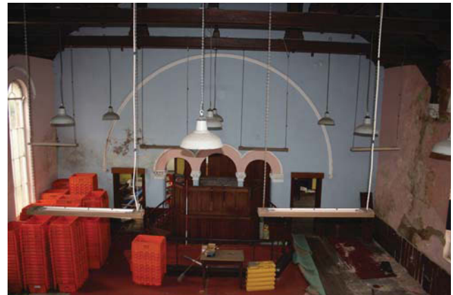
Plate 16. Chapel, pulpit from balcony, looking south, Scale: 2m.
