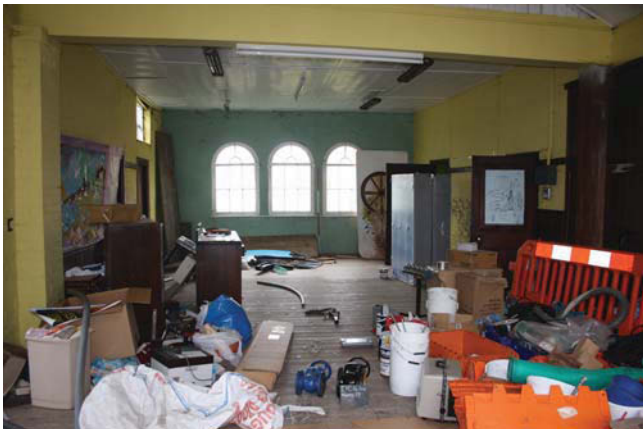
Plate 23. Sunday School hall, looking west, Scales: 2m and 1m.
