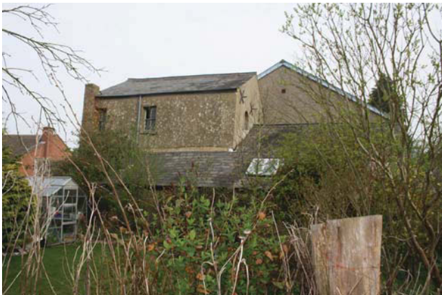
Plate 11. Exterior, rear elevation, looking north.
