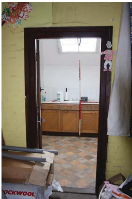
Plate 27. Kitchen, looking south, Scales: 2m and 1m.
