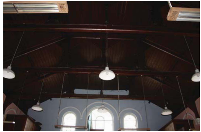
Plate 20. Chapel, roof trusses, looking north.
