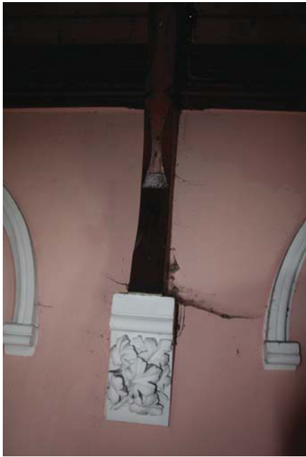
Plate 21. Chapel, truss support detail, west wall.
