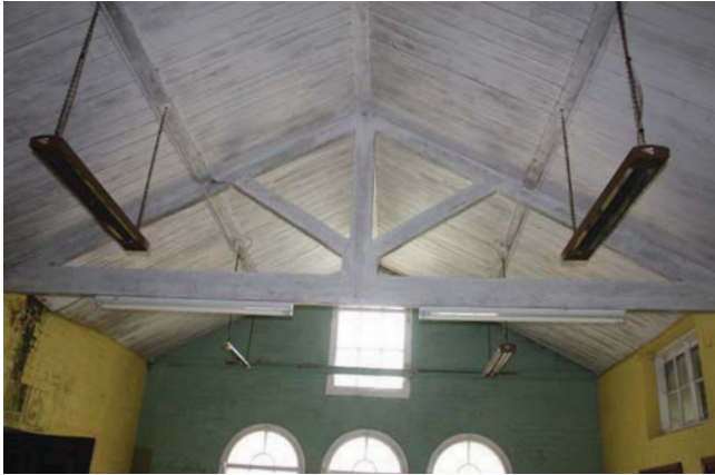
Plate 25. Sunday School, roof truss, looking east.
