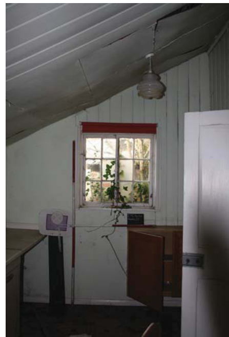
Plate 28. Office, looking west, Scales: 2m and 1m.
