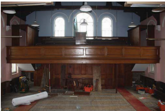
Plate 15. Chapel, rear looking at balcony, looking north, Scales: 2m and 1m.
