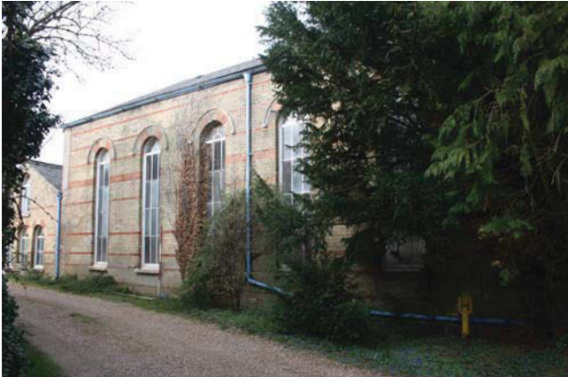
Plate 9. Exterior, East elevation, north end.
