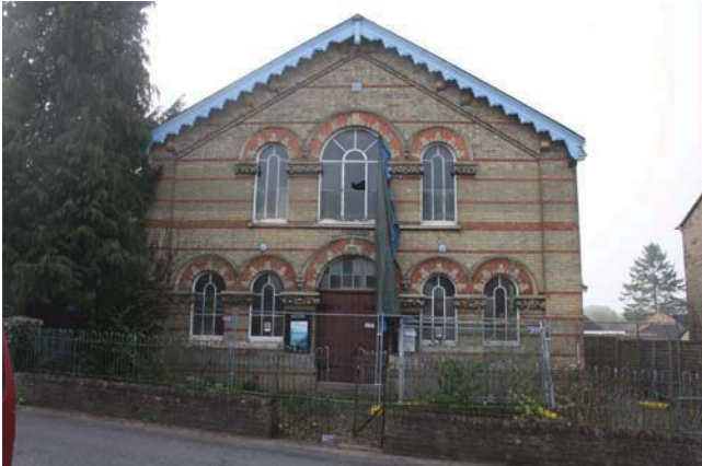
Plate 1. Exterior, front elevation, looking south, Scale 2m.
