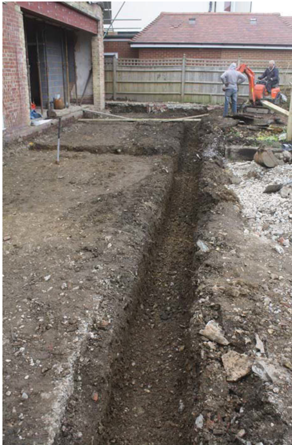
Plate 1. General view of new footing, looking north.
