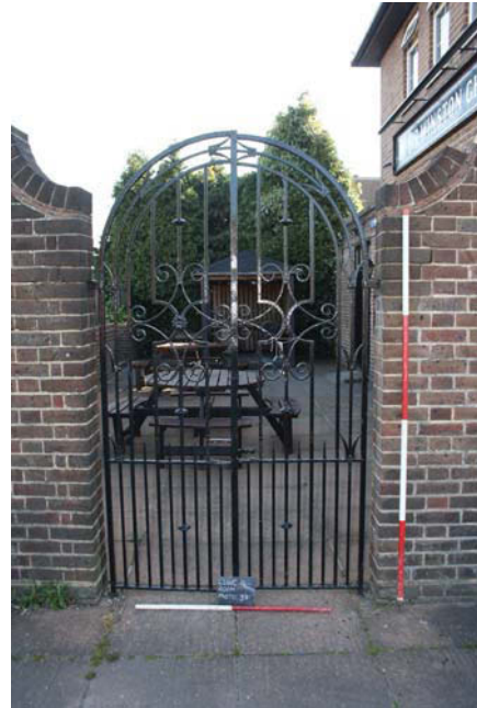
Plate 6. Exterior looking NE – Detail of gate Scales: 1m and 2m
