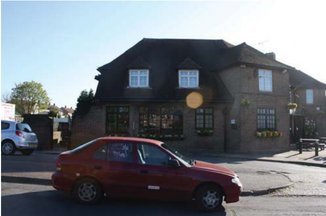
Plate 5. Exterior looking SE – General shot
