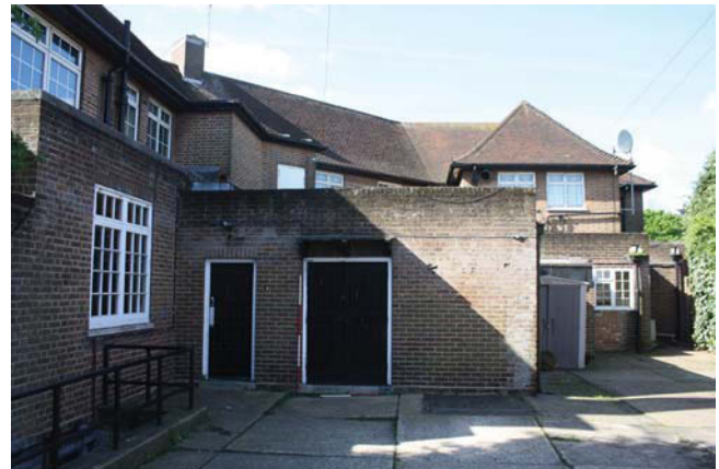
Plate 8. Exterior looking SW – General shot Scales: 1m and 2m
