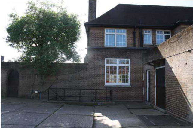
Plate 9. Exterior looking SE – General shot towards stairs Scales: 1m and 2m
