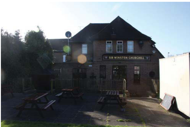
Plate 7. Exterior looking SE –General shot
