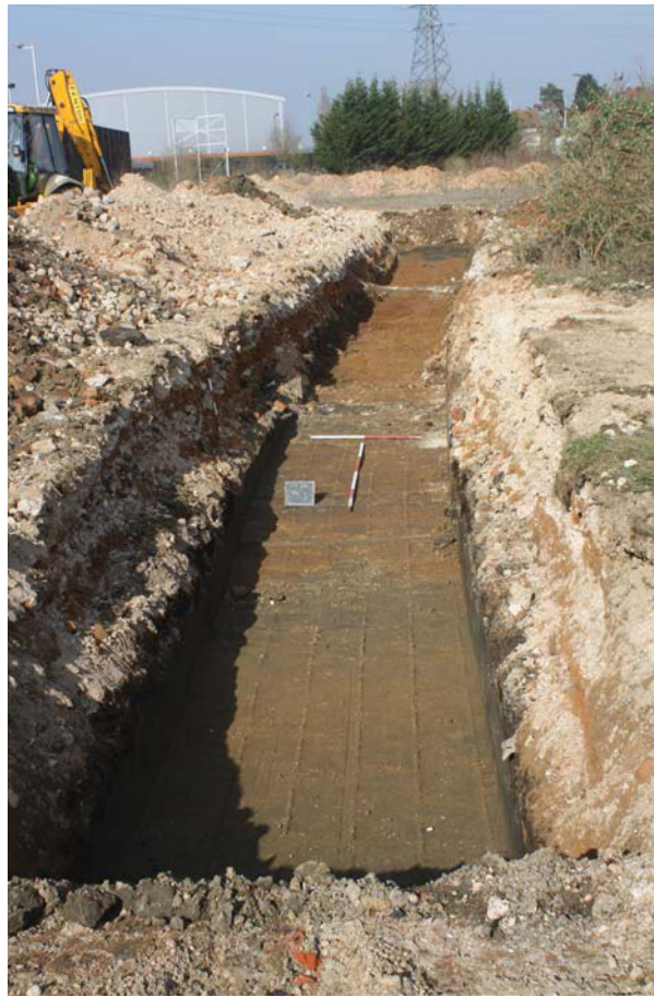
Plate 1. Trench 4, looking north, Scales: 2m and 1m.
