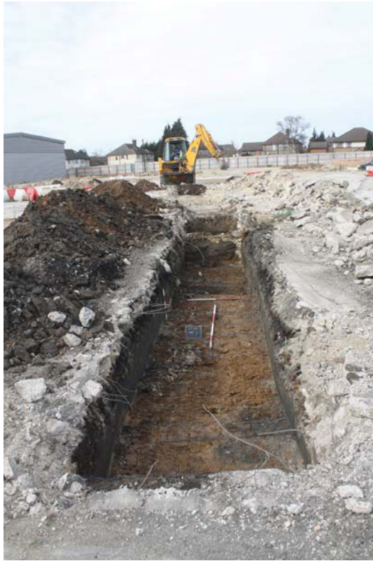
Plate 9. Trench 8, looking north, Scales: 2m, 1m and 0.5m.
