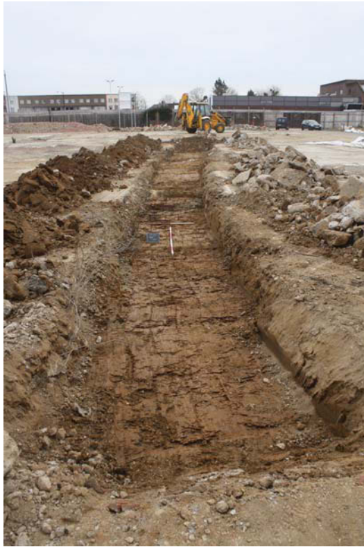
Plate 7. Trench 5, looking east, Scales: 2m, 1m and 0.5m.
