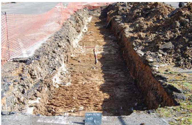
Plate 5. Trench 23, looking north, Scales: 2m, 1m and 0.3m.
