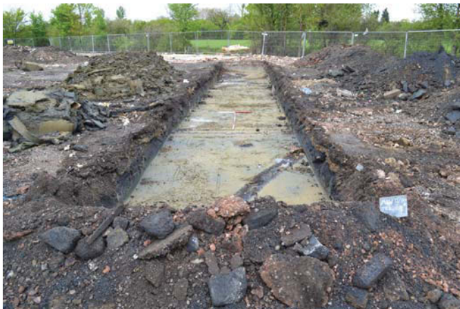
Plate 3. Trench 2, looking north, Scales: 2m, 1m and 0.3m.
