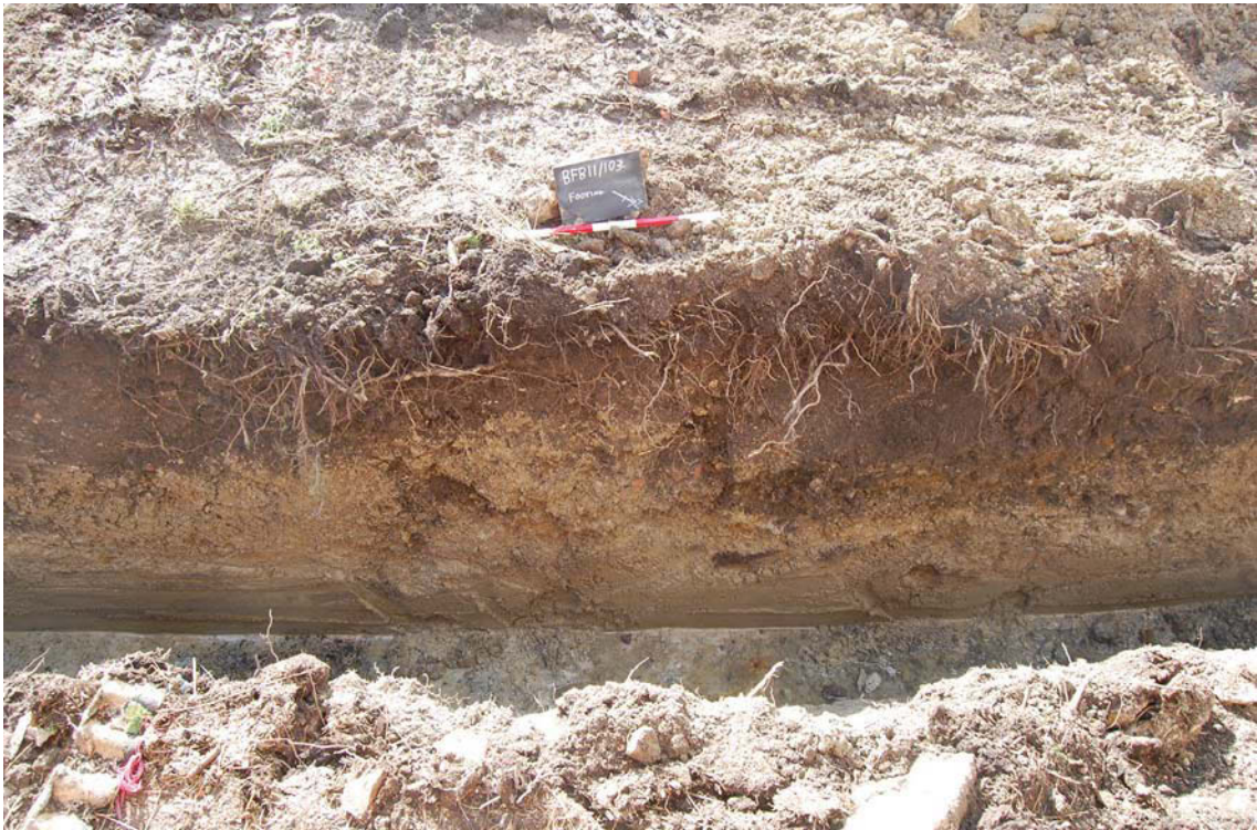
Plate 2. New footing, looking south east, Scale: 0.5m.
