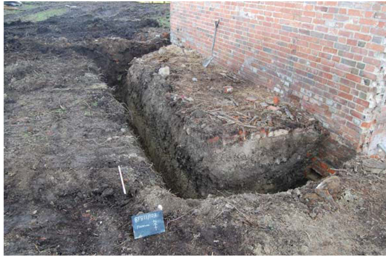
Plate 3. New footing trench, looking north, Scale: 0.5m.
