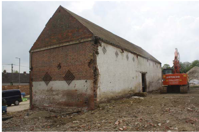
Plate 4. Barn during refurbishment, looking south, Scales: 2m and 1m.
