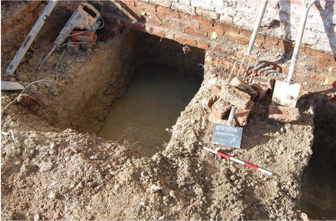
Plate 1. Underpinning trench, looking north, Scales: 0.5m.
