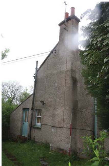
Plate 3. Gable end, looking northeast, Scales: 2m and 1m.
