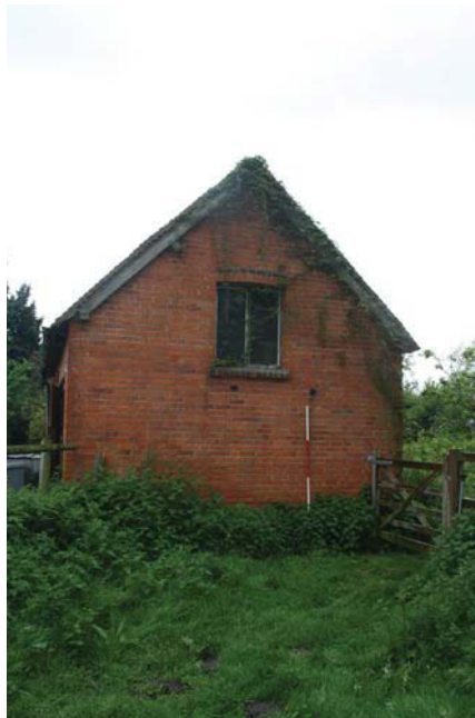
Plate 15. Gable end of barn, looking southwest, Scale: 2m.
