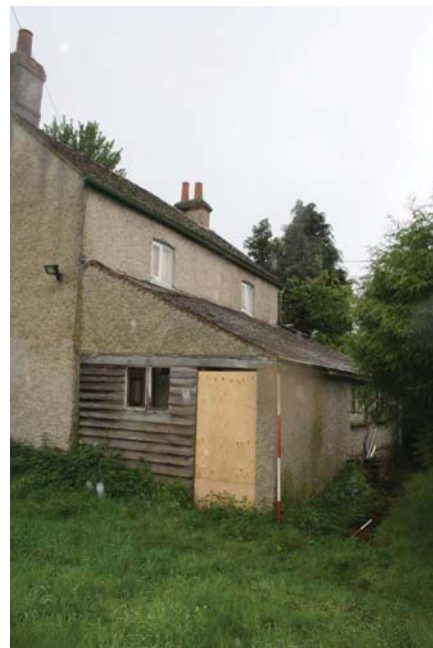
Plate 4. Rear elevation, looking southwest, Scales: 2m and 1m.
