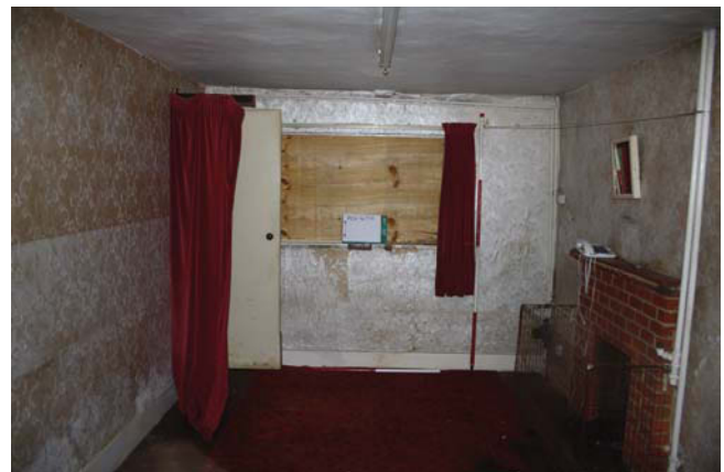
Plate 8. Room 2, looking southeast, Scales: 2m and 1m.
