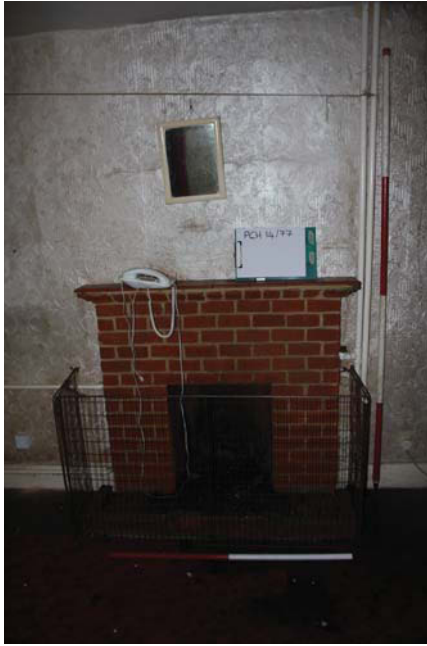
Plate 9. Fireplace in room 2, looking southwest, Scales: 2m and 1m.
