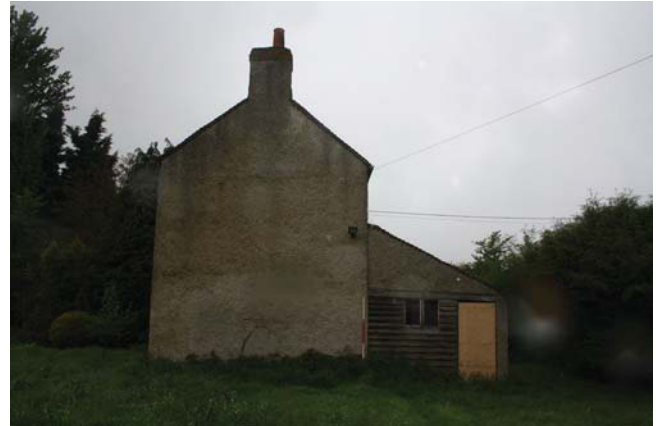
Plate 2. Gable end, looking southwest, Scales: 2m.
