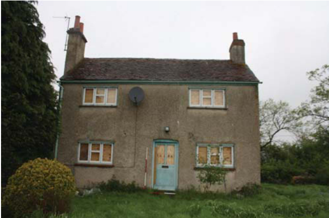
Plate 1. Front elevation, looking northwest, Scales: 2m and 1m.
