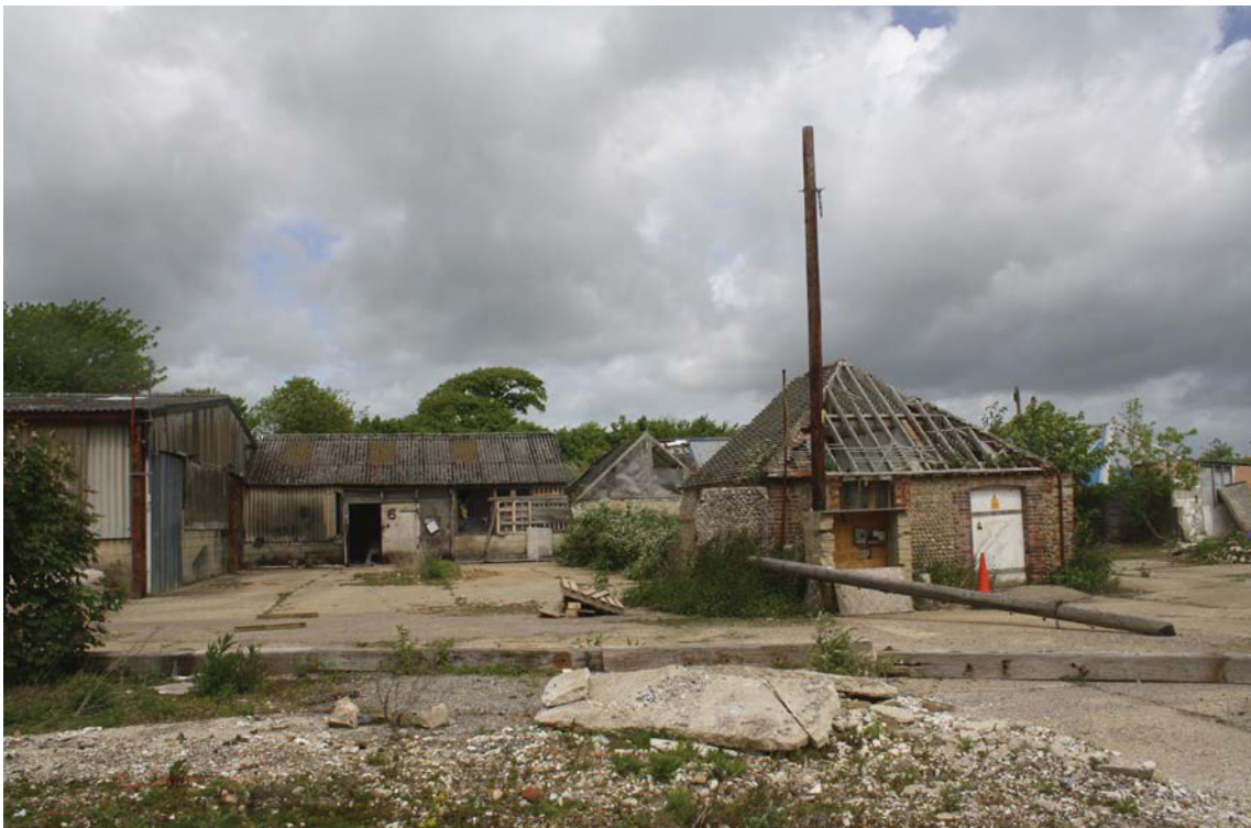
Plate 4. Buildings 3 and 4, looking north.
