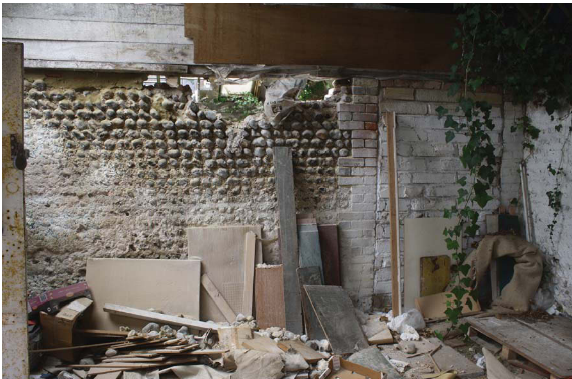
Plate 12. Interior of western wall of Building 5b, looking west.
