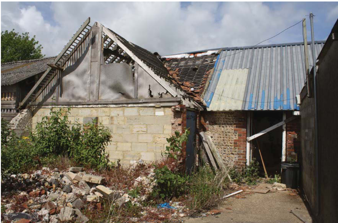
Plate 10. Buildings 5a and 5b, looking north.
