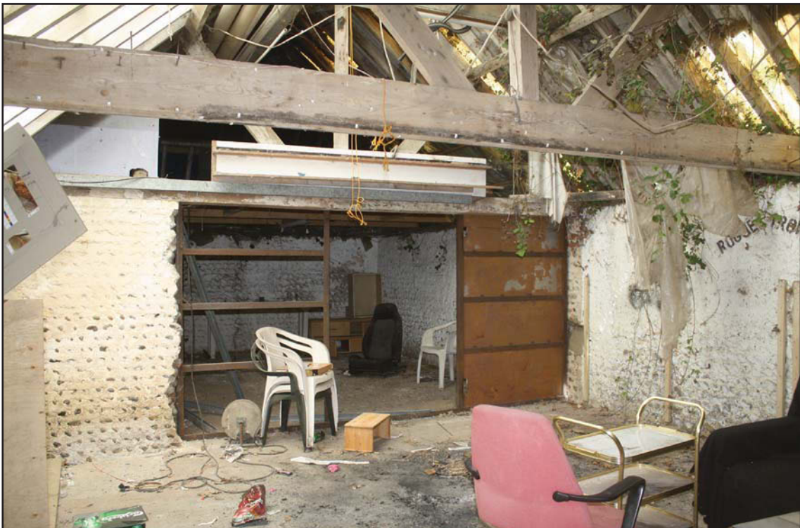
Plate 16. Interior of Building 5e, looking north.
