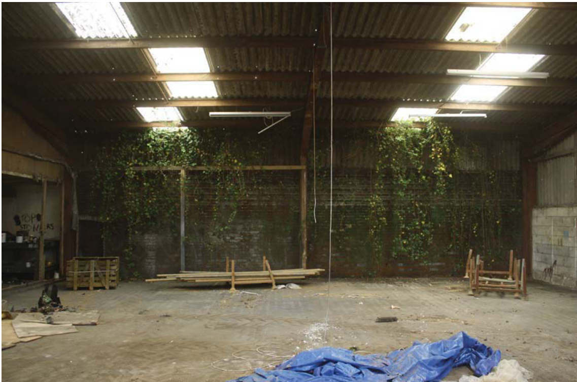
Plate 3. Interior of Building 1b, looking north.
