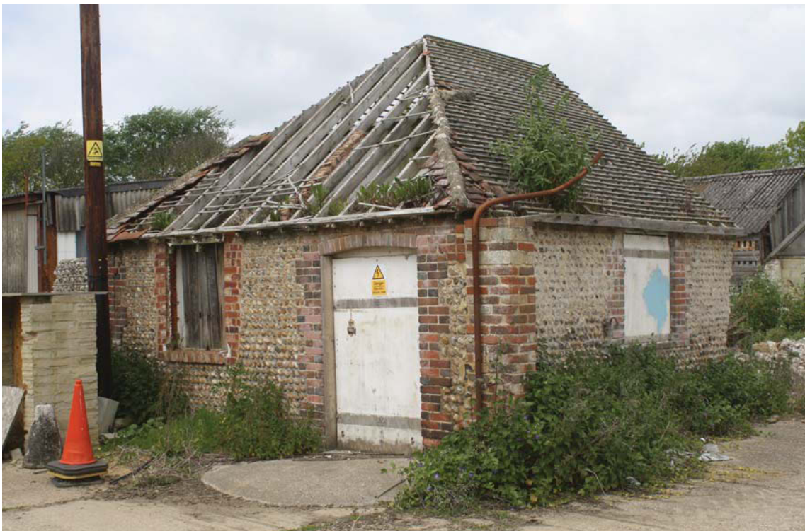
Plate 6. Building 4, looking north-west.
