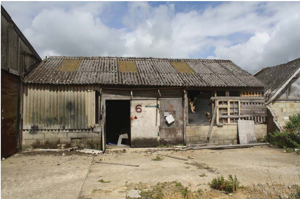
Plate 9. Building 3, looking north.
