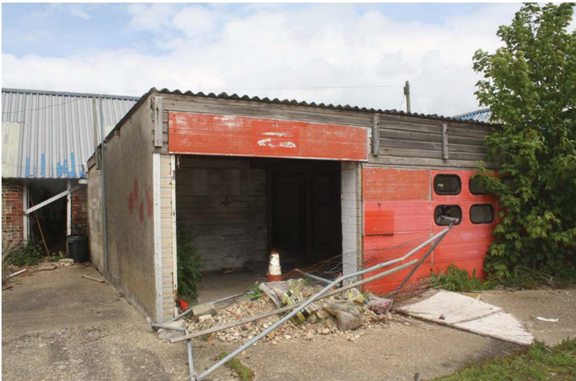
Plate 14. Building 7, looking north.
