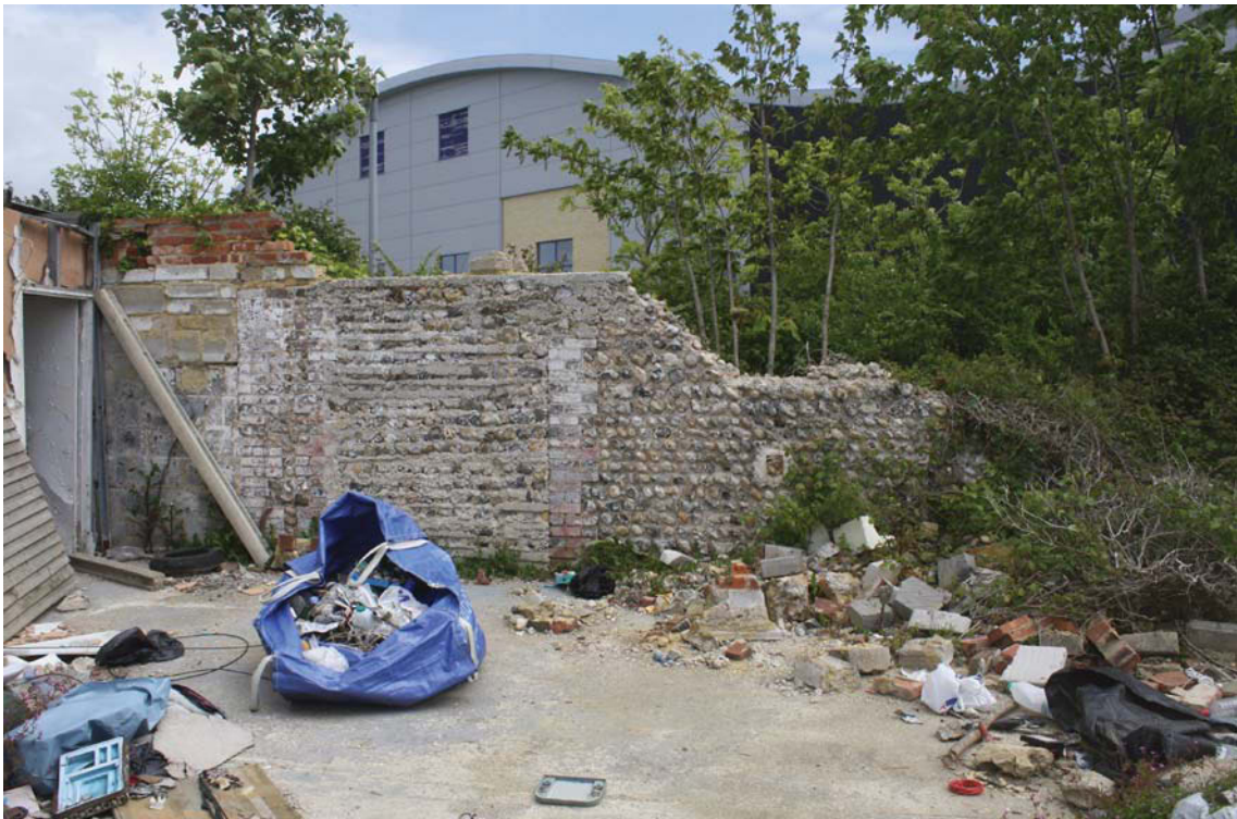
Plate 15. Demolished building at eastern end of site, looking east.
