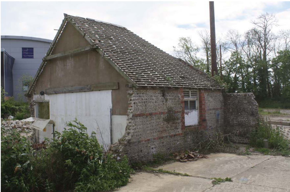
Plate 8. Rear of Building 4, looking south-east.
