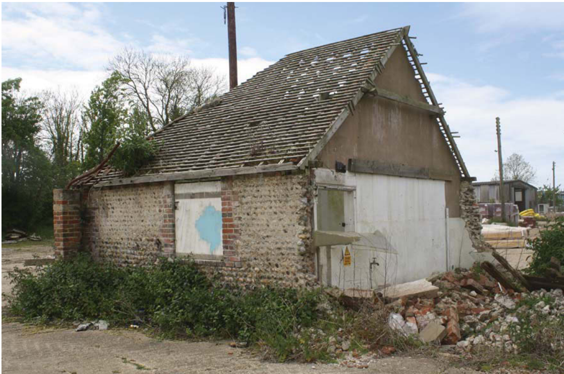
Plate 7. Rear of Building 4, looking south-west.
