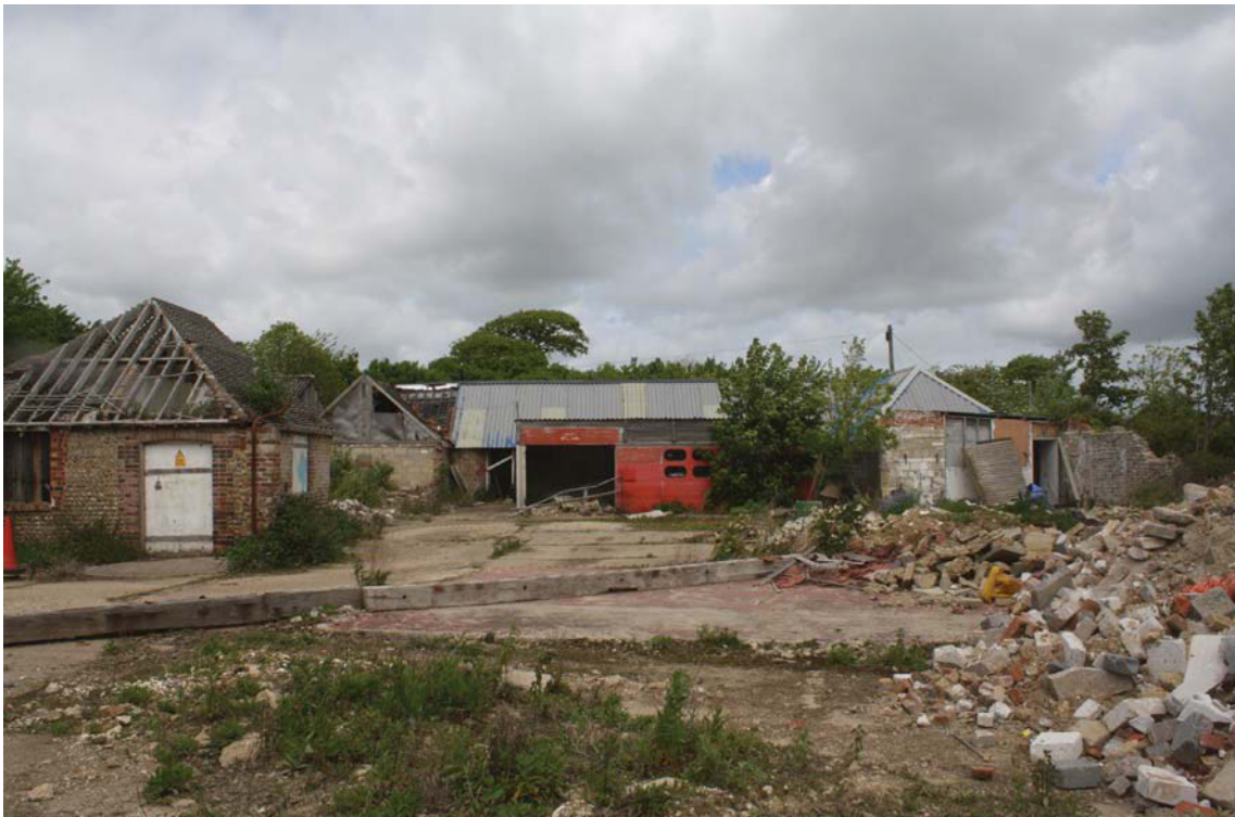
Plate 5. Building 7 with demolished area in foreground, looking north.
