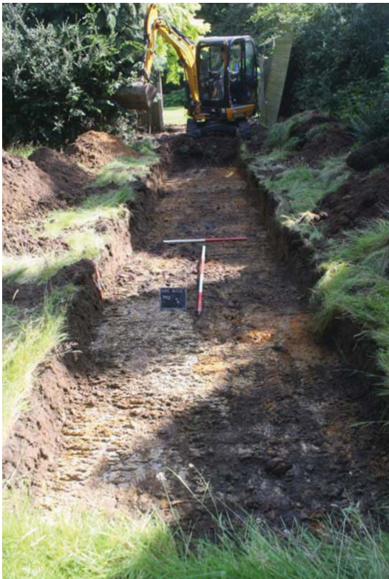
Plate 2. Trench 2, looking north east, Scales: horizontal 2m and 1m, vertical 0.3m.
