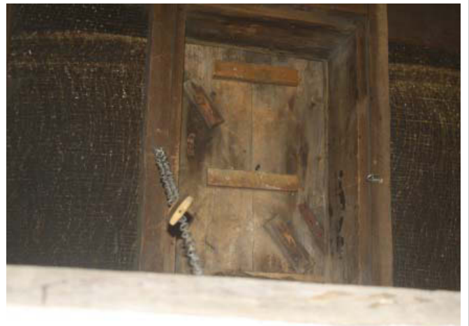
Plate 8. Interior, southern loft, hatch to exterior of roof, looking NE
