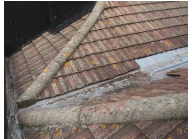
Plate 4. Exterior, roof, detail of western gutter and parapet, looking NNE
