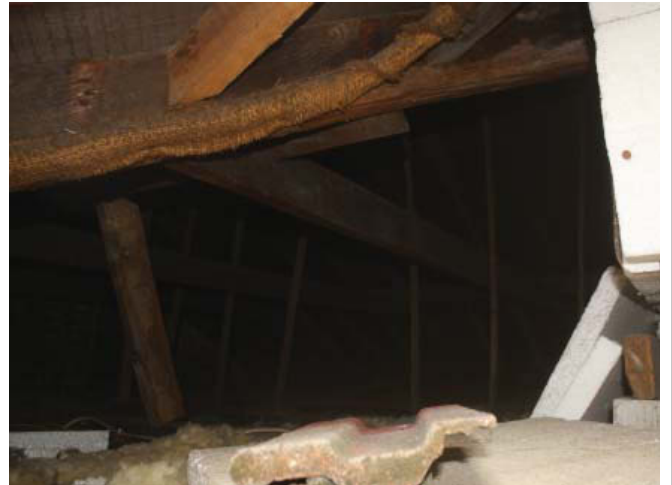
Plate 6. Interior, southern loft, looking ENE
