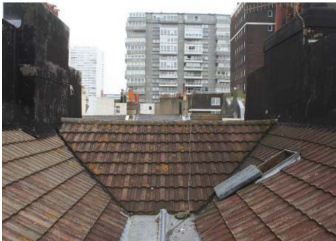
Plate 3. Exterior, roof, general view, looking ESE
