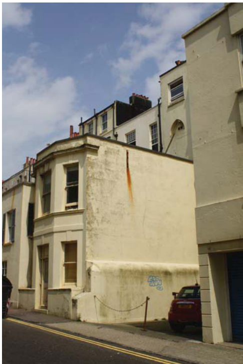
Plate 27. Exterior, Montpelier Road, general view looking ENE
