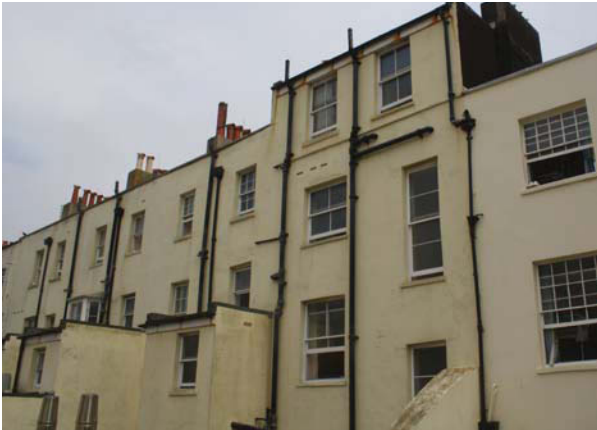
Plate 21. Exterior, rear of 33 Oriental Place and adjacent properties to north, looking ENE from roof terrace
