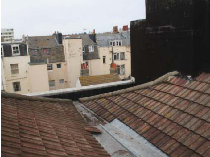
Plate 1: Exterior, roof, general view, looking NW
