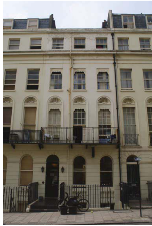
Plate 26. Exterior, Oriental Place, 33 Oriental Place, looking WNW
