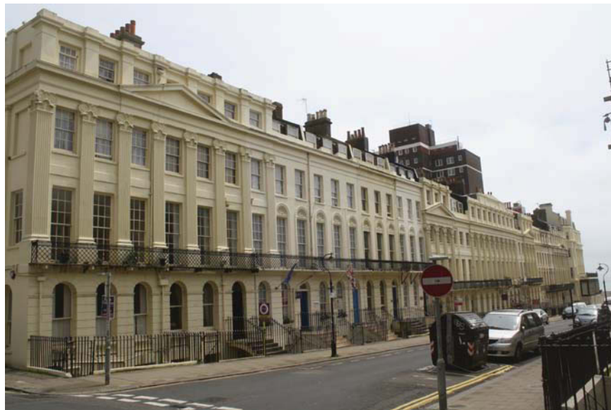
Plate 30. Exterior, Silwood Street, Oriental Place (east terrace), looking South
