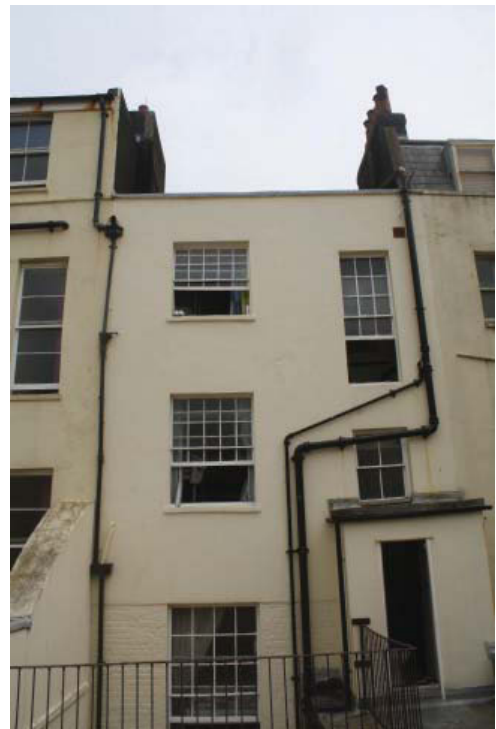
Plate 20. Exterior, rear of 33 Oriental Place, looking ESE from roof terrace
