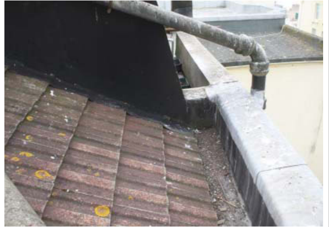
Plate 2. Exterior, roof, western gutter and parapet, looking SSW
