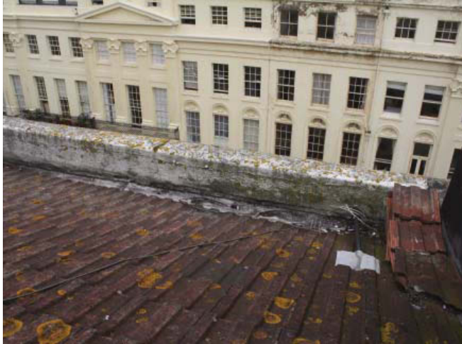
Plate 5. Exterior, roof, view of eastern gutter and parapet, looking ESE
