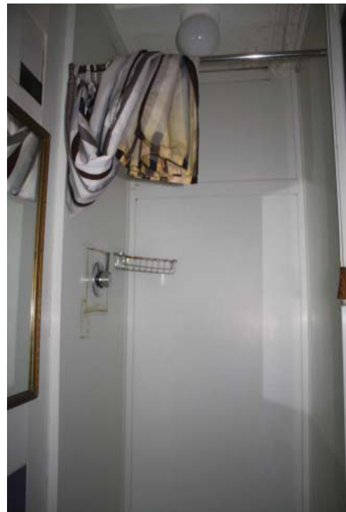
Plate 12. Interior, shower room C, looking WNW
