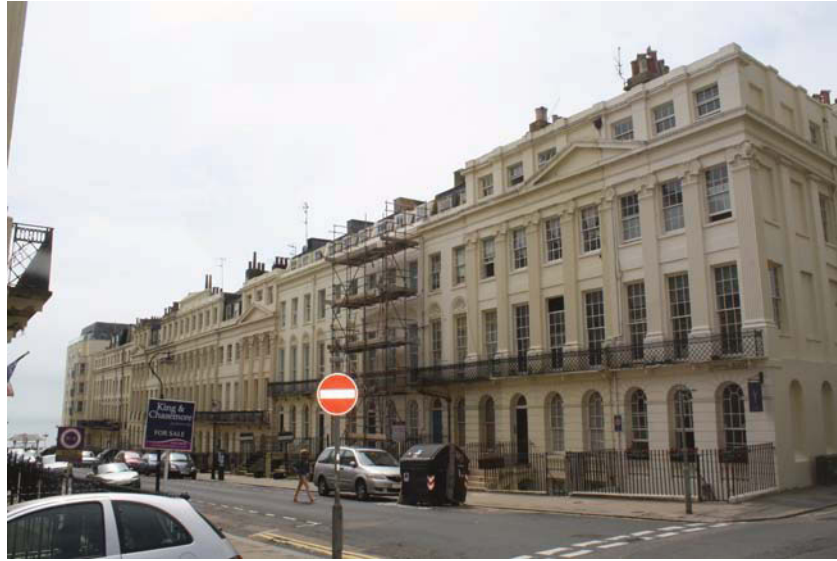
Plate 29. Exterior, Silwood Street, Oriental Place (west terrace), looking SW
