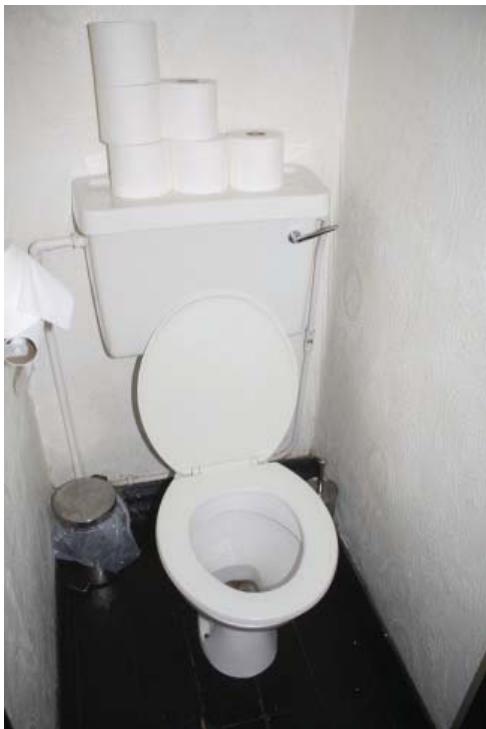
Plate 11. Interior, WC B, looking SSW
