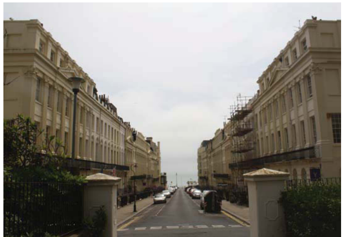
Plate 28. Exterior, Silwood Street, general view looking SSW towards Oriental Place
