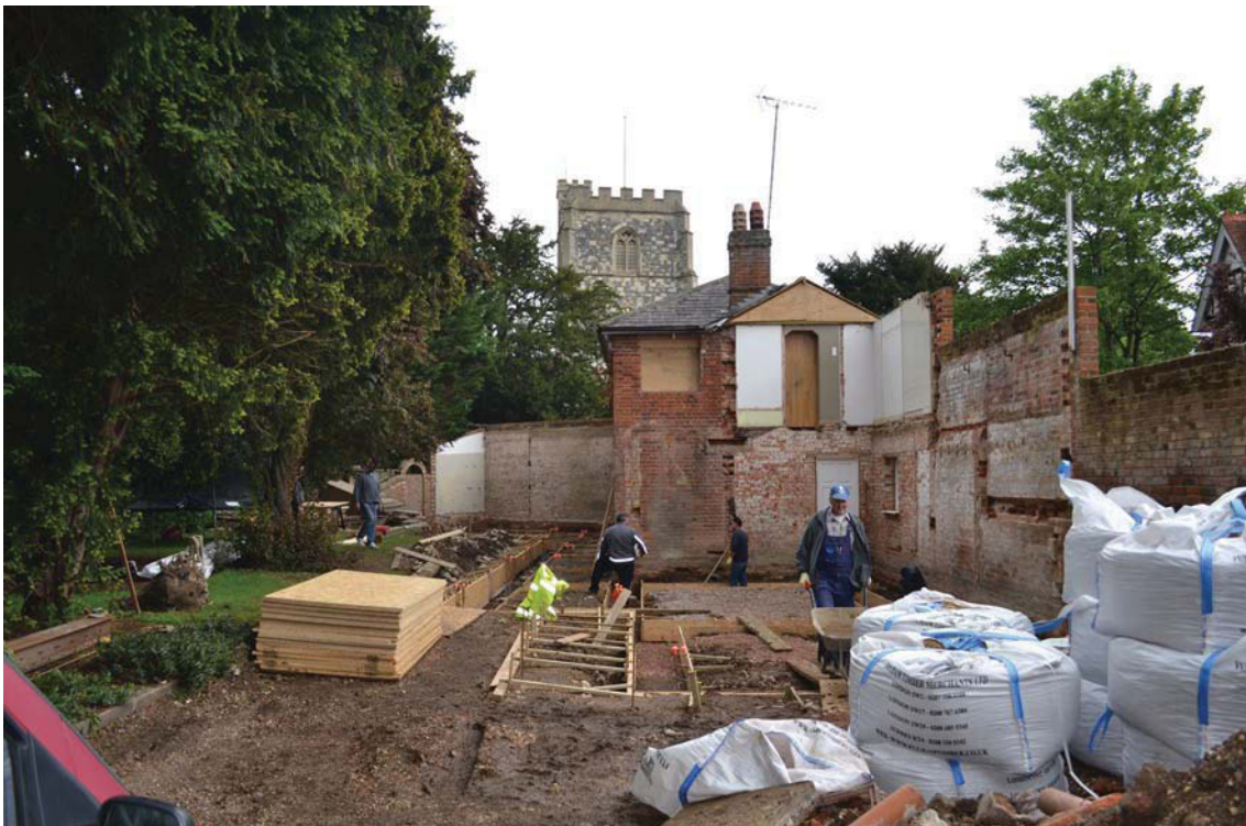
Plate 2. Site showing reduced dig.
