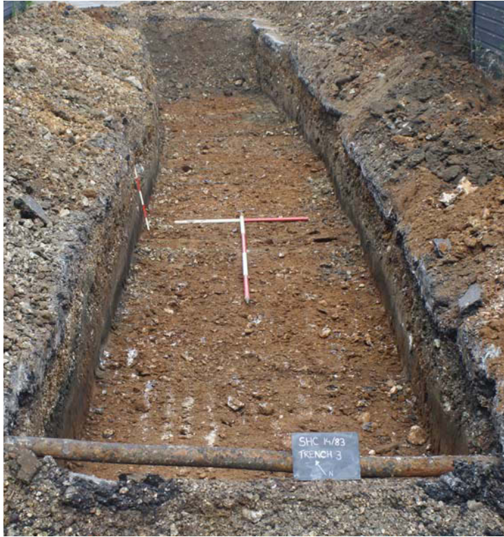
Plate 3. Trench 3, looking north east, Scales: 2m, 1m and 0.5m.
