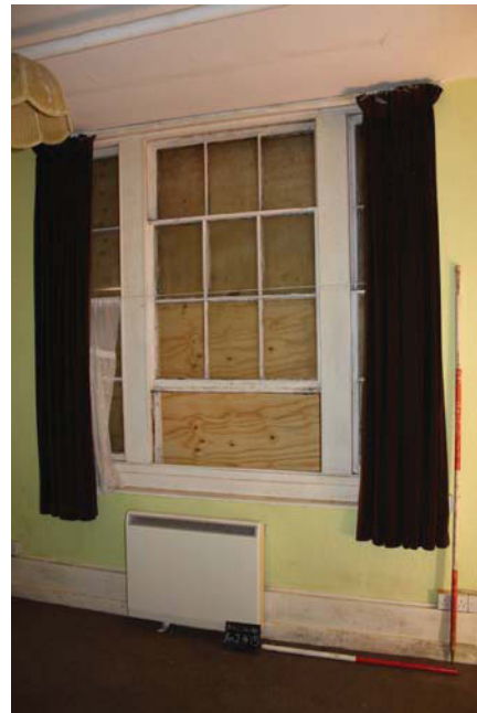
Plate 8. Flat 4 Room 2, Window detail, looking E, Scales: 1x1m 1x2m.
