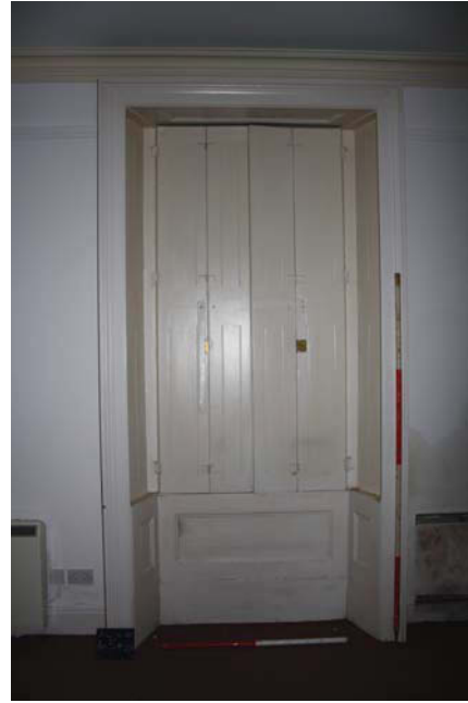
Plate 14. Flat 5 Room 6, Shutter window detail, looking NW. Scales: 1x1m 1x2m.
