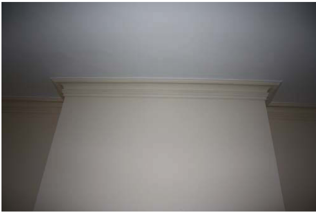
Plate 15. Flat 5 Room 7, Ceiling detail, looking NW.
