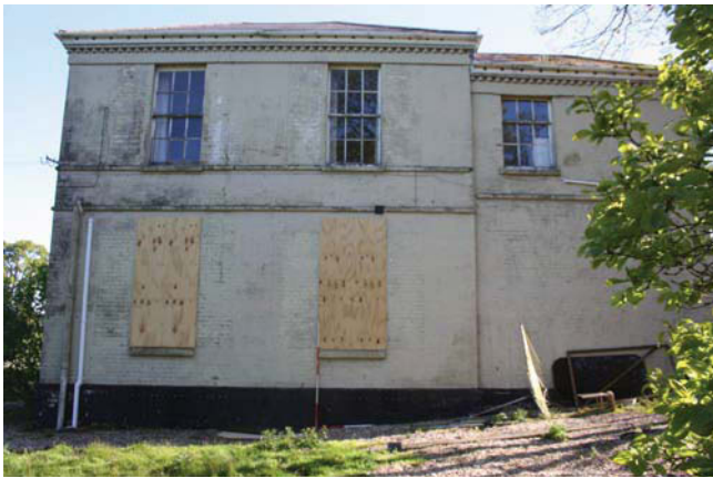
Plate 3. SW face of house, looking NE. Scales: 1x1m 1x2m.
