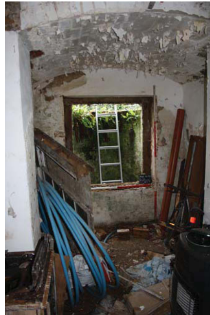
Plate 6. Cellar Room 26, General shot and light-well, looking NW, Scales: 1x1m 1x2m.
