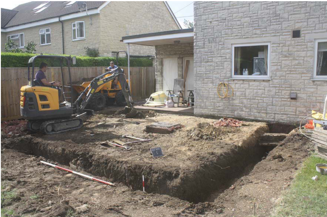
Plate 1. New footings, looking south, Scales:2m.
