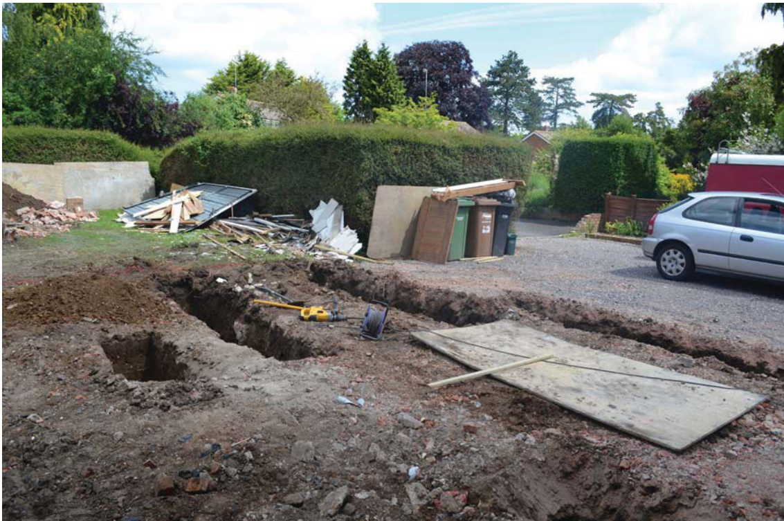
Plate 1. Area of new footings, looking north east.
