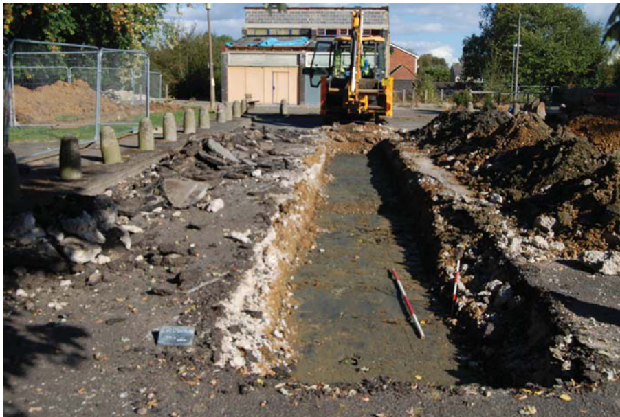
Plate 5. . Trench 1, looking east, Scales: 2m and 0.5m.
