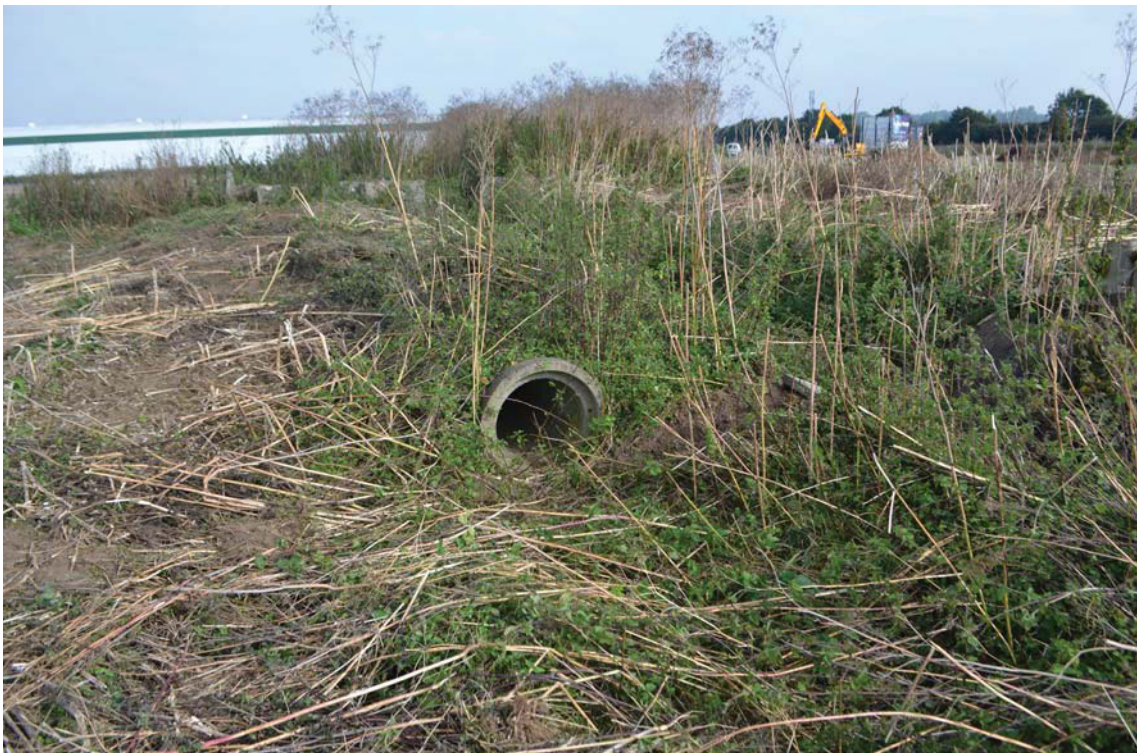
Plate 2. Exposed concrete culvert, looking north north east.
