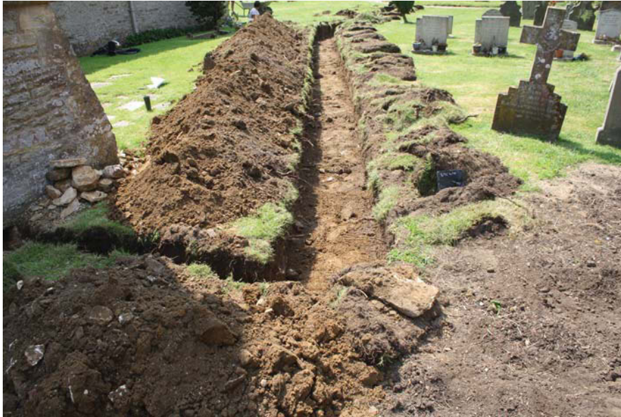
Plate 1. View of trench, looking west.
