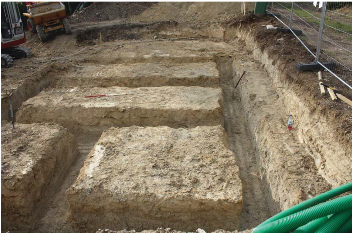
Plate 2. View over excavated footing, looking west, Scale: 1m.
