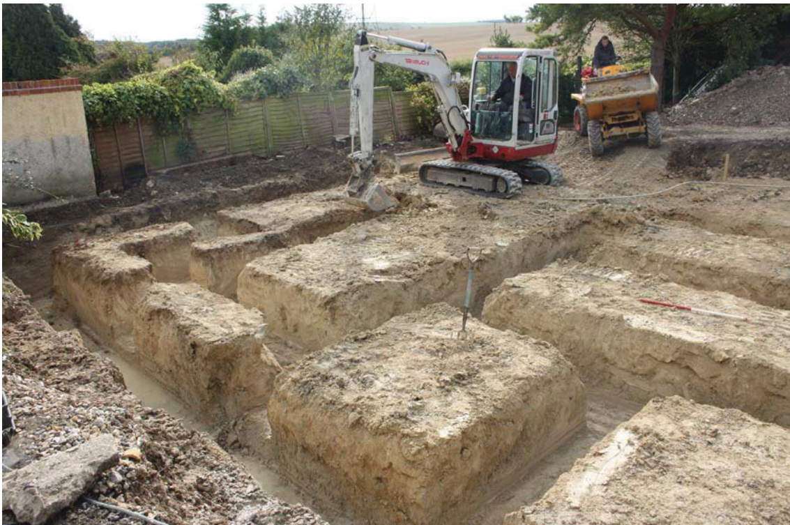
Plate 1. View over excavated footings, looking south west, Scale: 1m.
