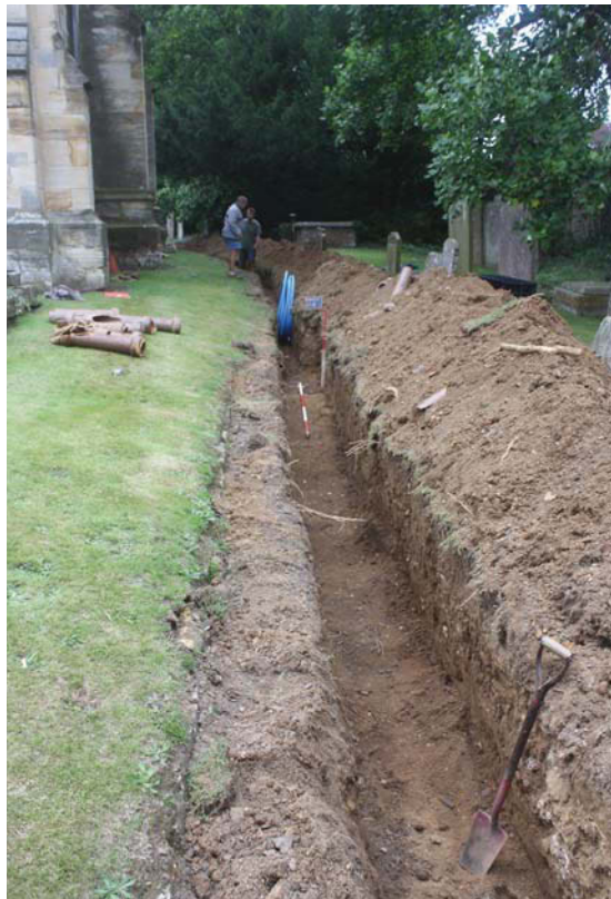
Plate 4. Pipe trench in east, looking north, Scales: horizontal 2m, vertical 1m.
