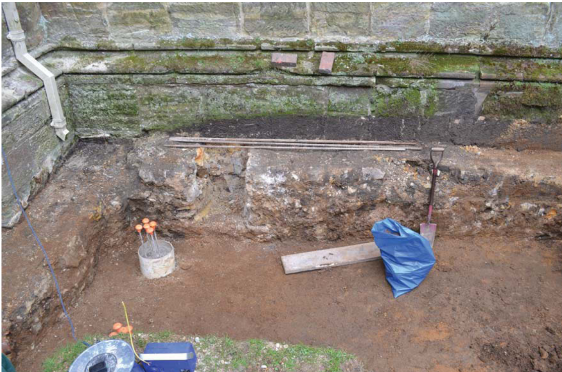
Plate 1. Church foundation in area of ground reduction looking south.
