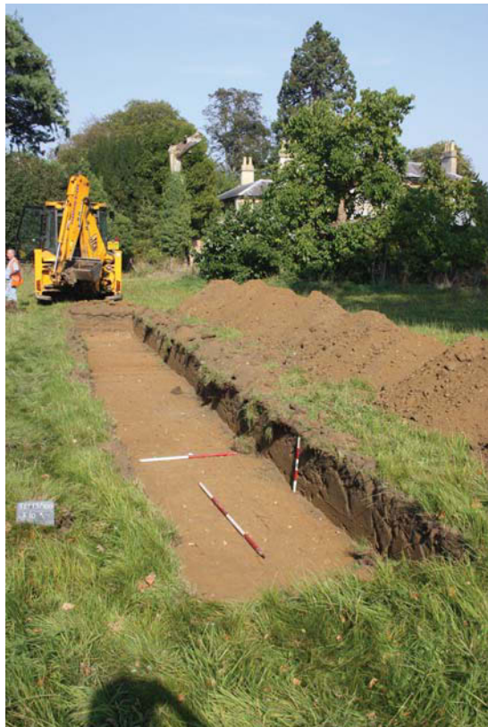
Plate 2. Trench 10, looking north east, Scales: horizontal 2m and 1m, vertical 0.5m.
