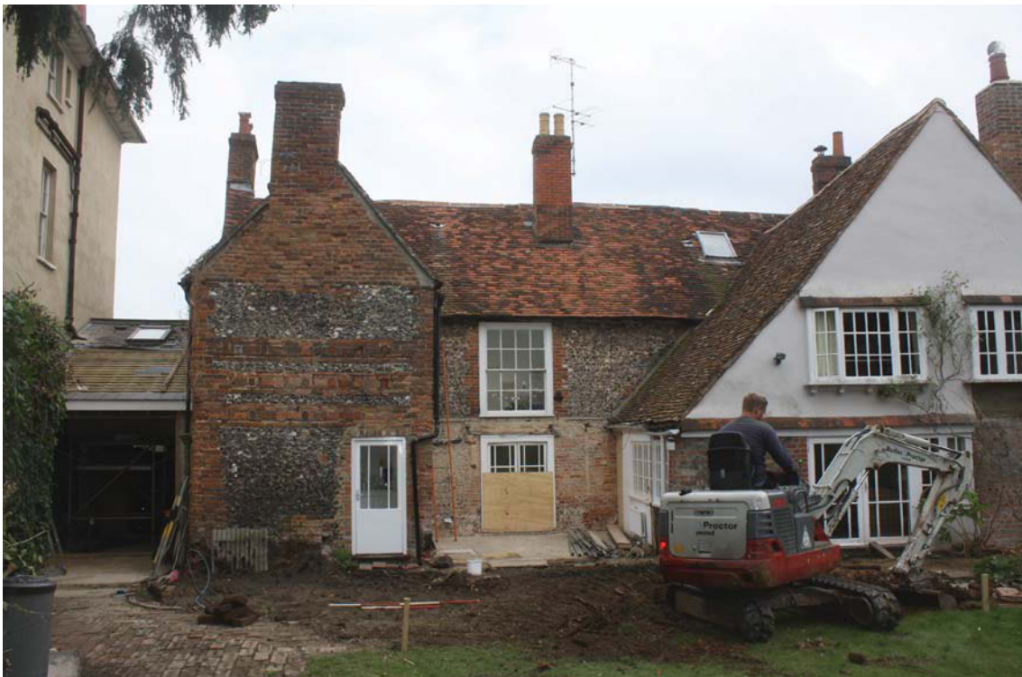
Plate 1. Ground reduction in progress, looking northeast, Scale: 2m.
