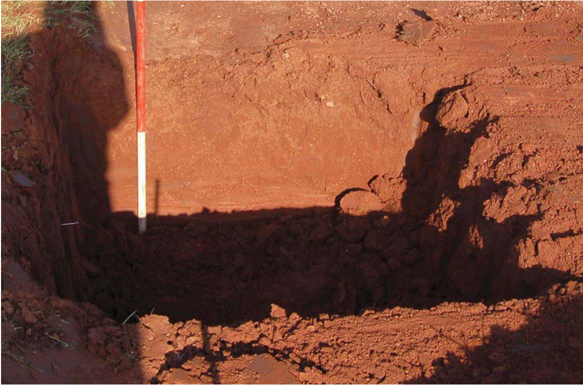
Plate 3. Stanchion pit 8, looking east-north-east (1m scale)
