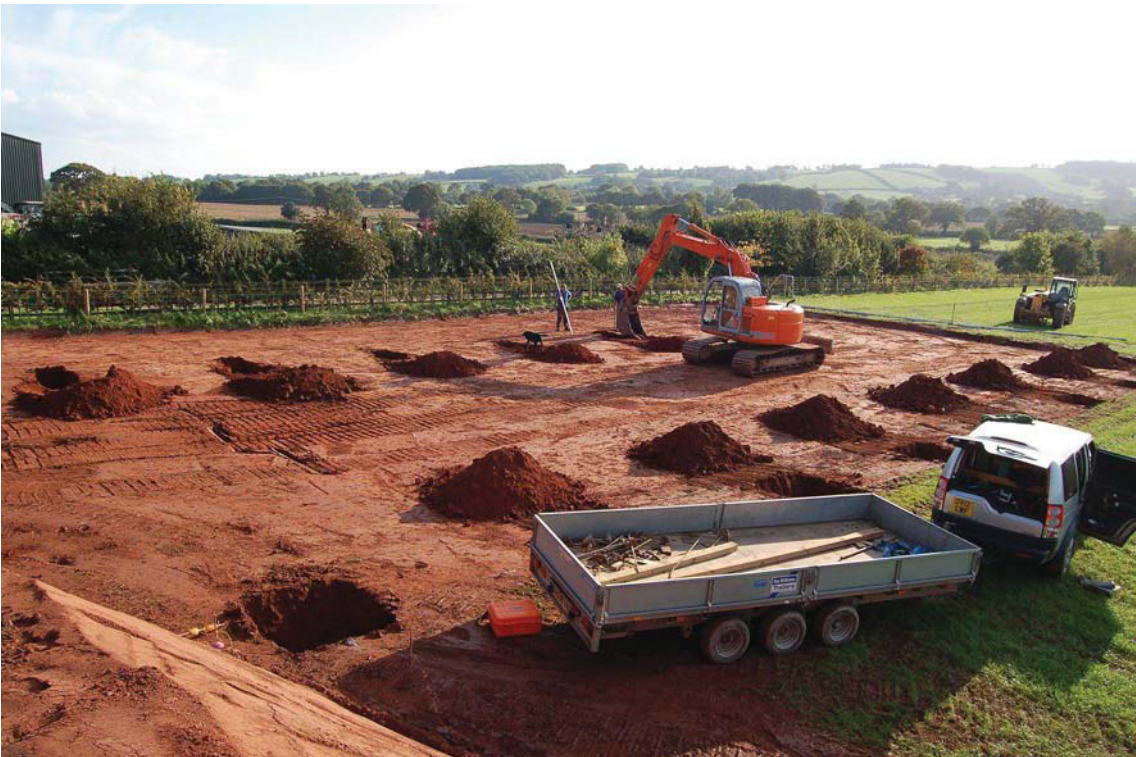
Plate 2. Excavation of the stanchion pits, looking south-west
