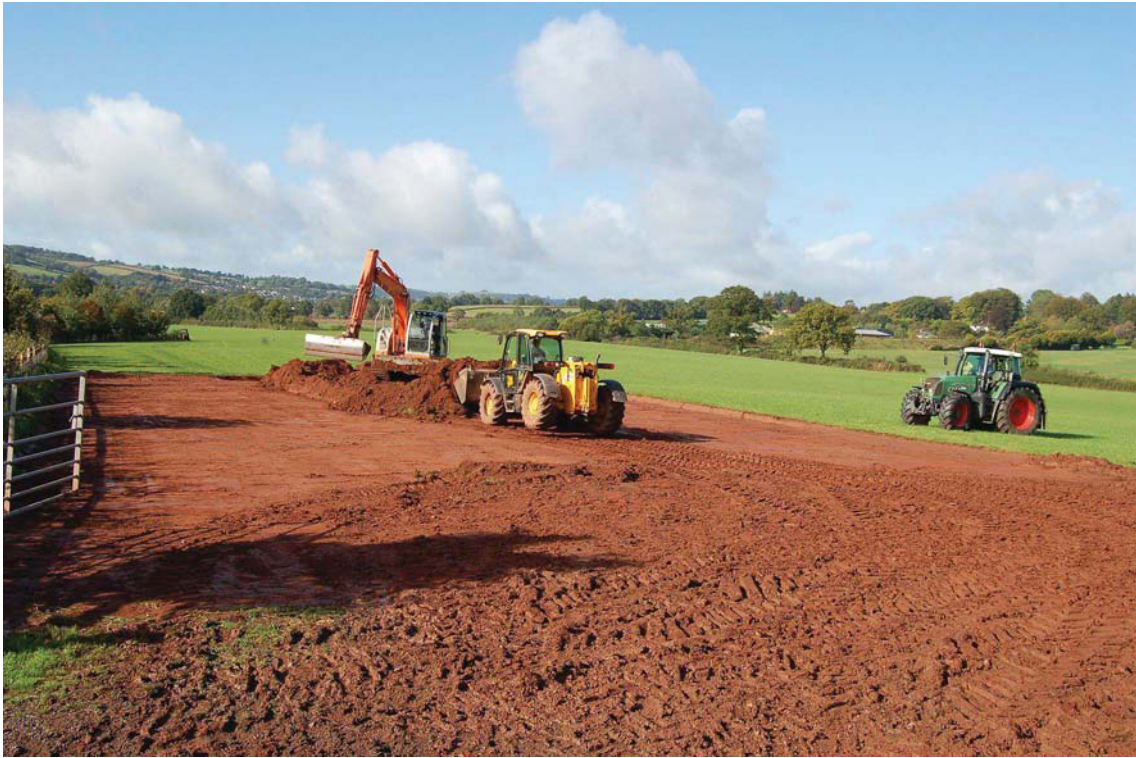
Plate 1. Stripping of the upper topsoil, looking west
