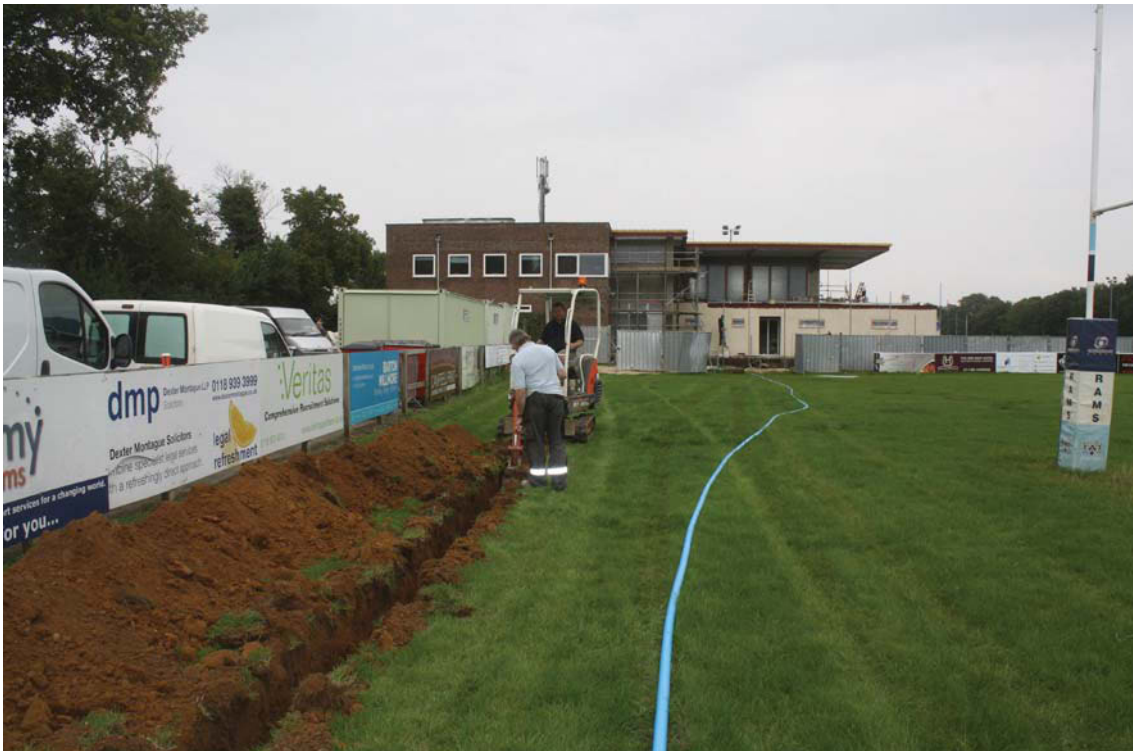
Plate 1. Pipe trench under excavation, looking north east.
