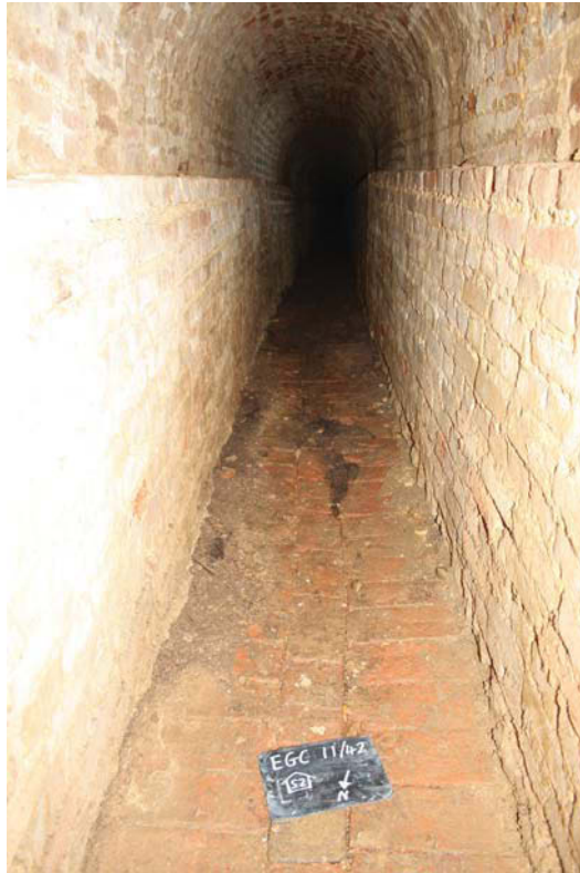
Plate 3. General view of tunnel, looking south from entry point
