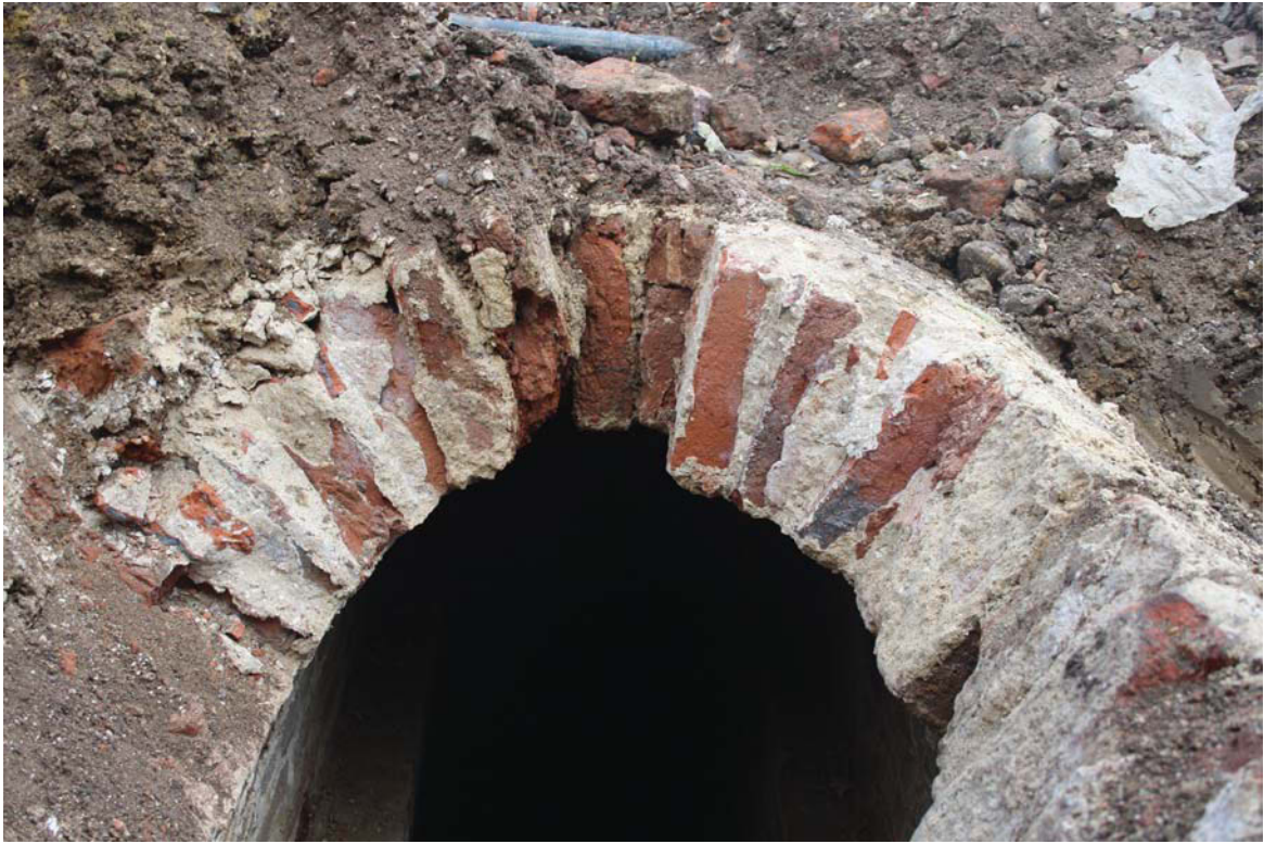
Plate 7. Detailed view of arched brickwork at opening
