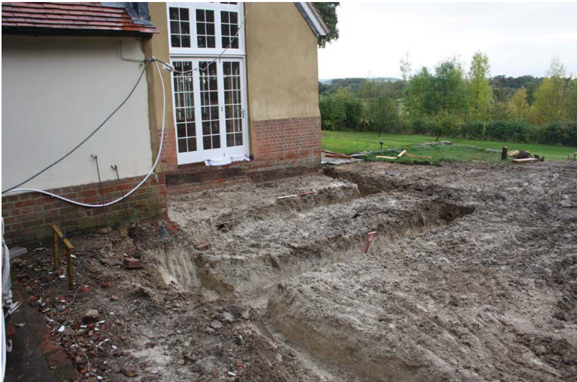
Plate 1. Location of watching brief, looking south west.
