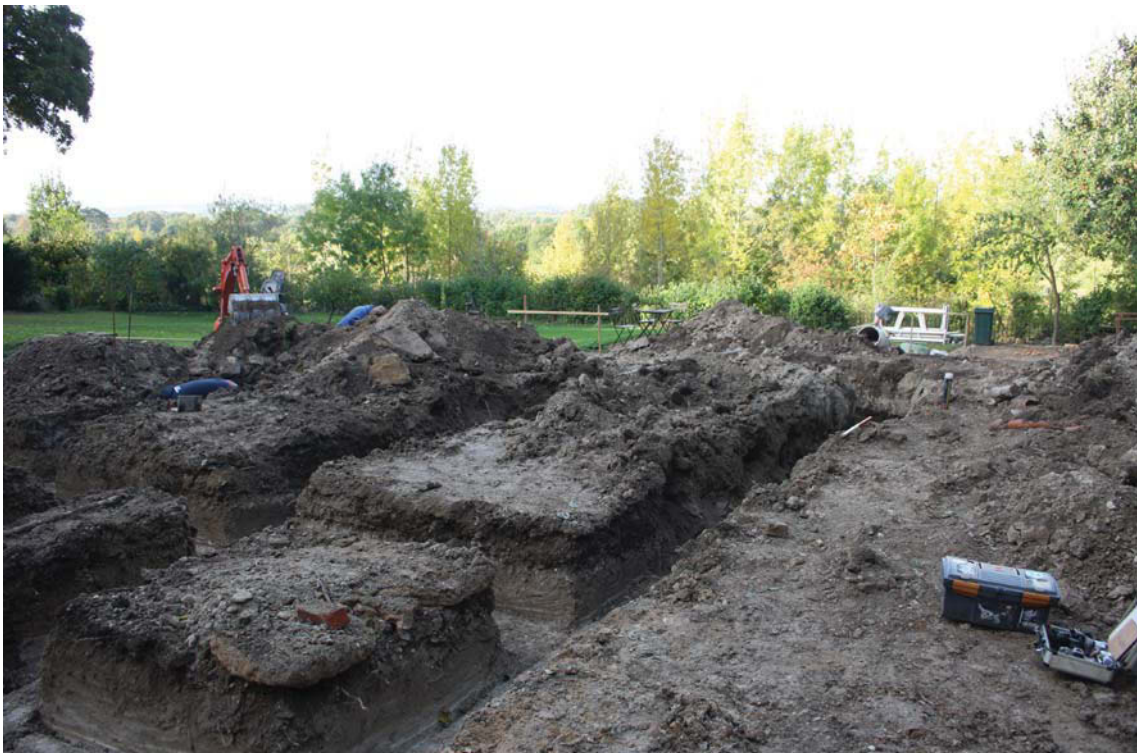
Plate 2. Footing trenches looking west.
