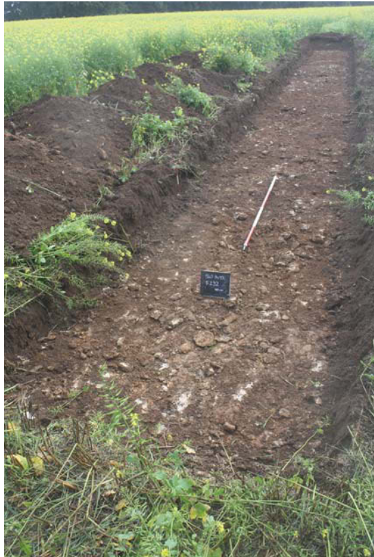
Plate 15. Trench 232, looking east, Scales: 2m and 0.30m.
