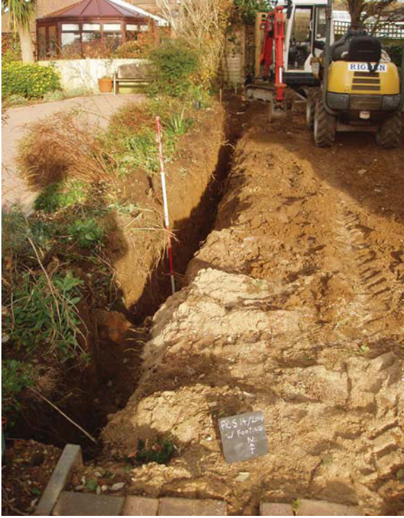
Plate 1. West footing looking north; Scale: 2m
