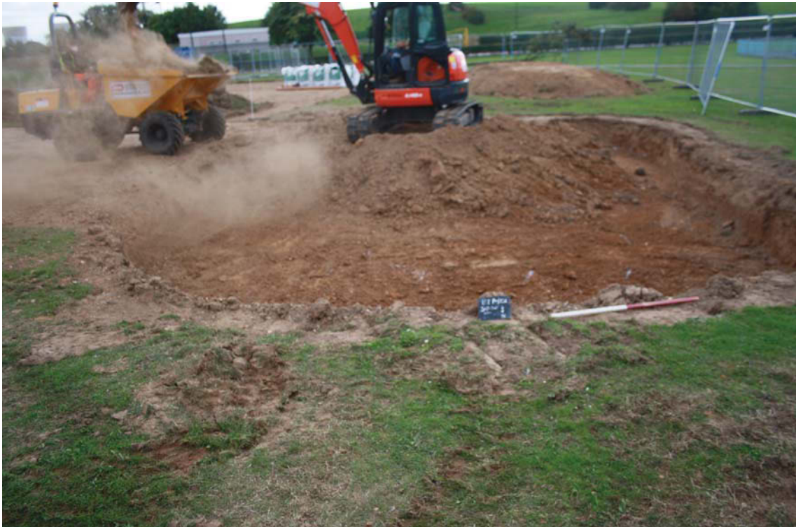
Plate 1. Skate bowl excavation, looking south, Scale: 1m.
