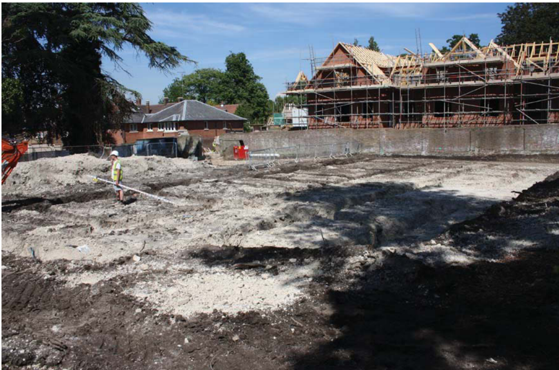
Plate 6. Site looking north-east
