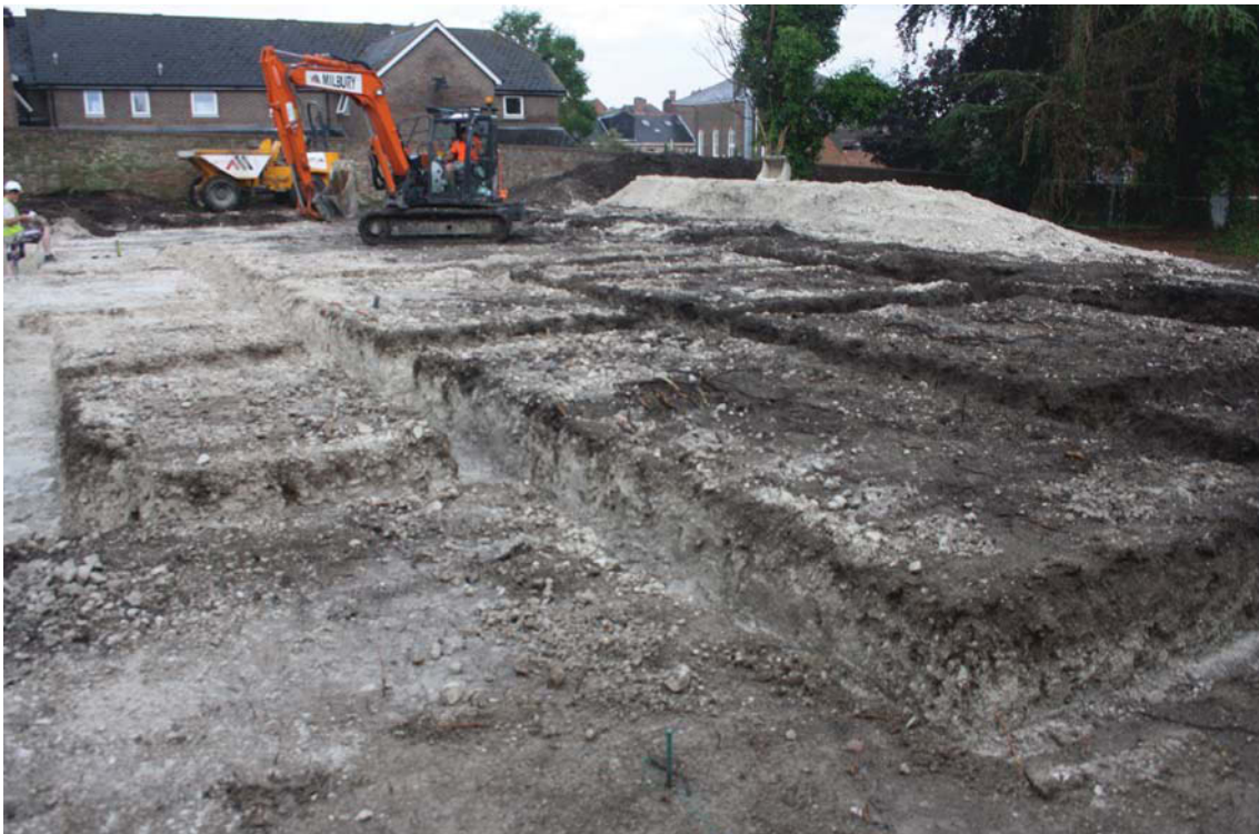
Plate 1. Footings, looking north-west, Scales: 2m and 1m.
