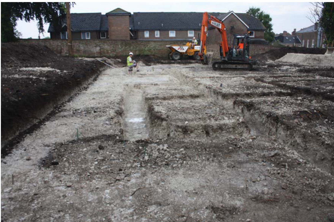
Plate 2. Footings, looking west.
