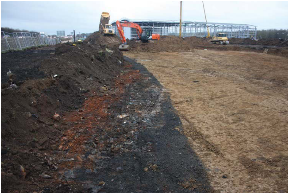
Plate 2. Modern truncation along east boundary of site, looking south.
