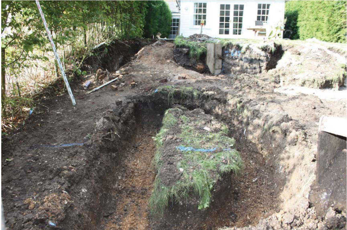
Plate 3. Planter footing, looking west.
